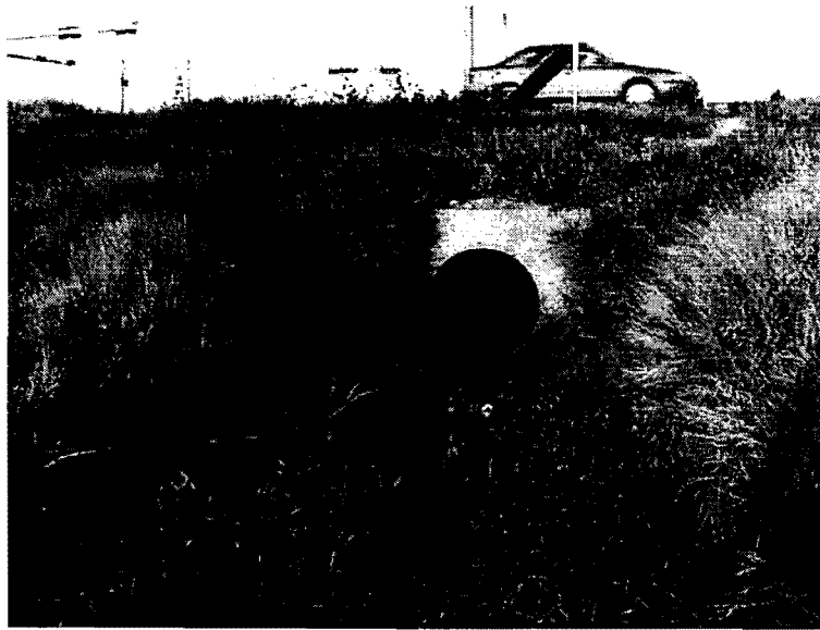
Figure 5.22 Safety End Treatment in Laredo District.
