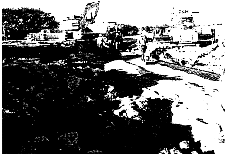
Figure 5.6 Pipe with Backfill up to the Crown.
