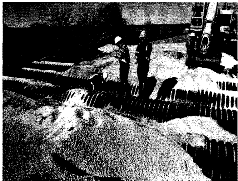
Figure 5.49 Wichita Falls Installation.
