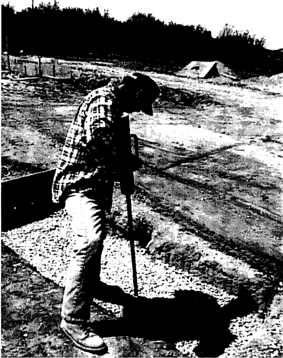
Figure 4.4. The Dynamic Cone Penetrometer Being Operated.
