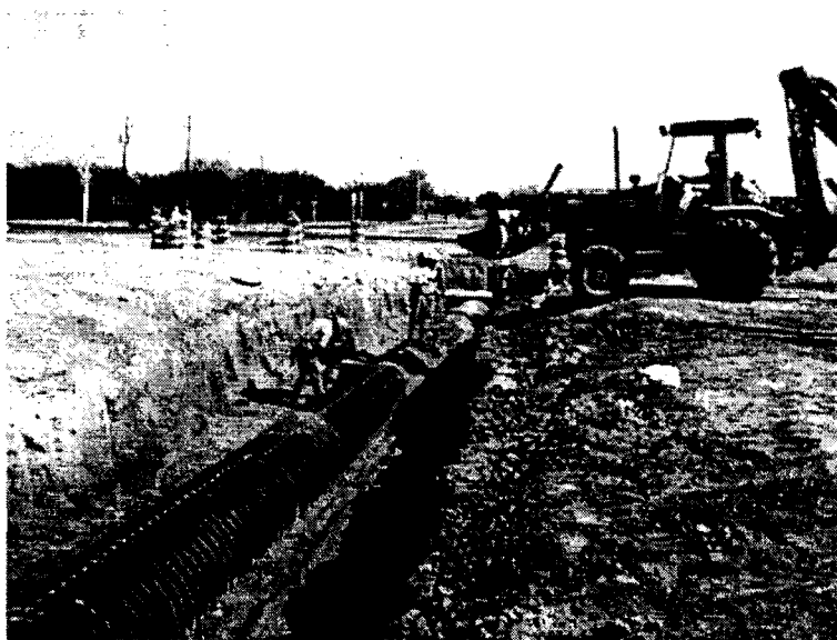
Figure 5.17 Backfill Placement and Compaction.
