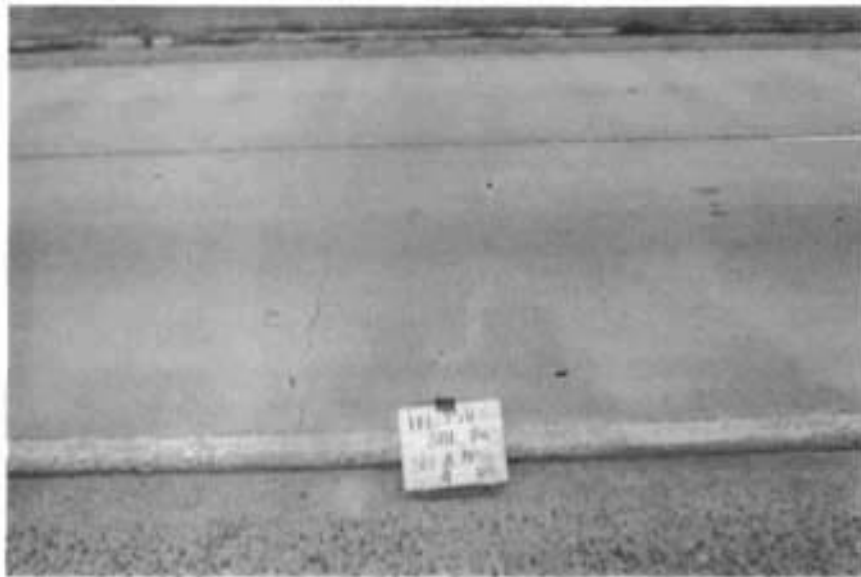
Fig A3.5 Typical minor transverse cracking, Johnson County.
