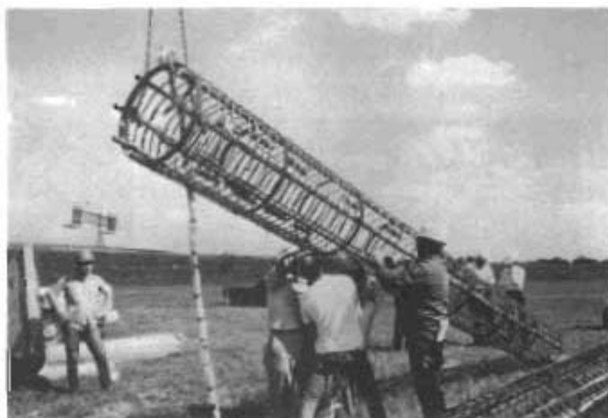
Fig 6.1. Manifold being tied to the steel cage for shaft MT1.
