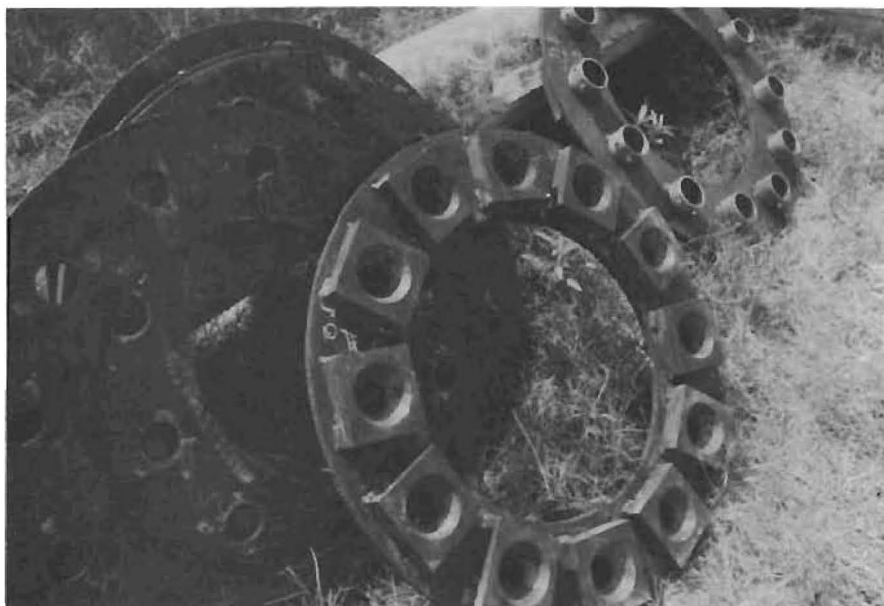
Fig 6.7. Two sides of the annular base plate used in the anchor shafts.
