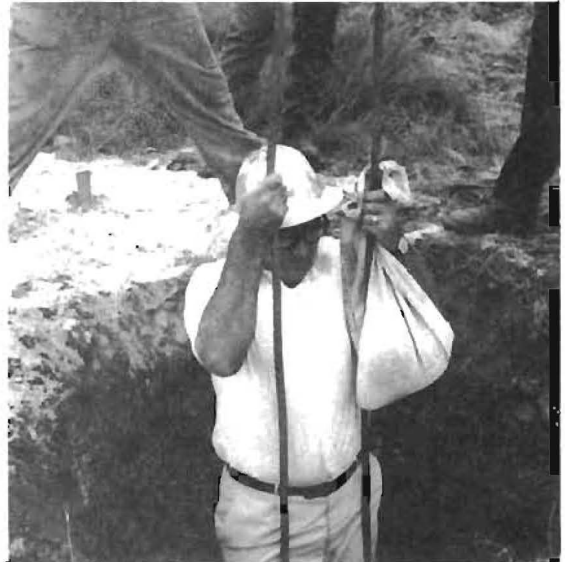
b. Manual Cleaning of the Bottom of a Dry Hole
