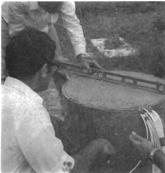
i. Forming of the Top Section of a Test Shaft
