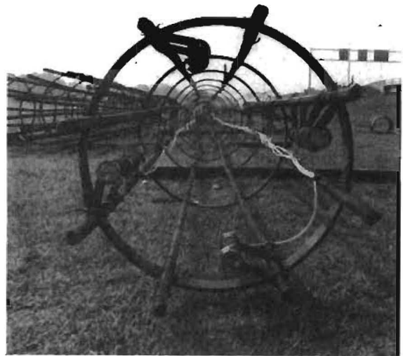
b. View from the Tip of the Instrumented Steel Cage
