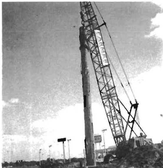
a. Extraction of the Shaft at G1 Site
