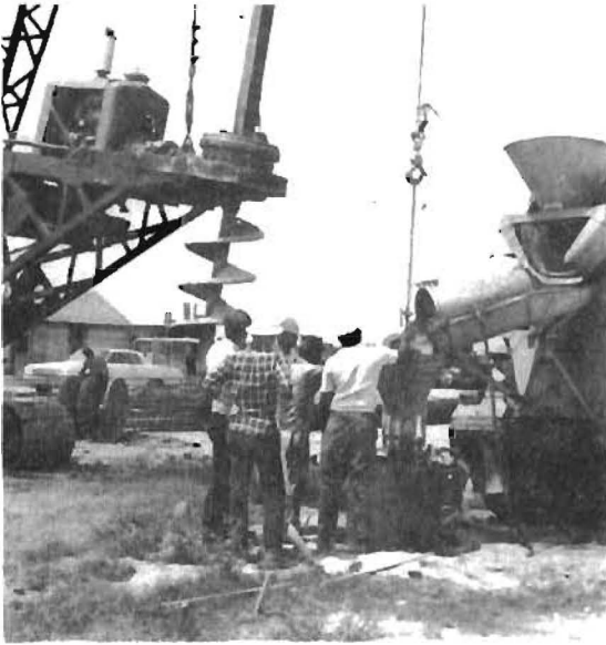
g. Concreting of a Dry Hole
