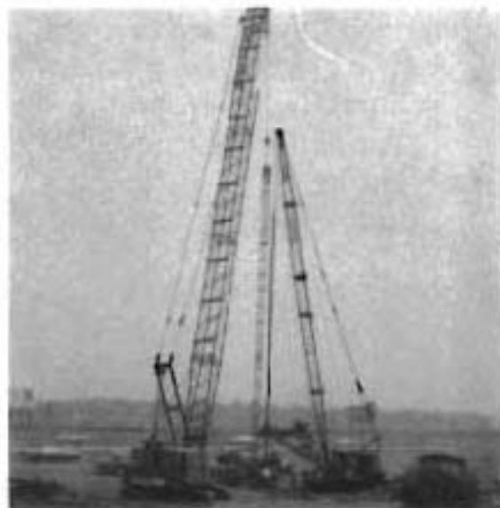
e. Installation of Steel Cage in the Hole
