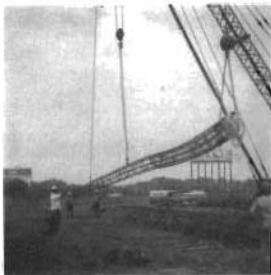
d. Lifting of Instrumented Steel Cage
