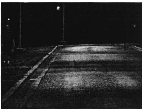
Figure 8.52 20% target image at the second target location on line 1.
