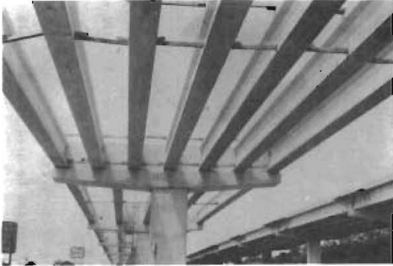
(a) Erected girders with temporary timber braces and tie downs
