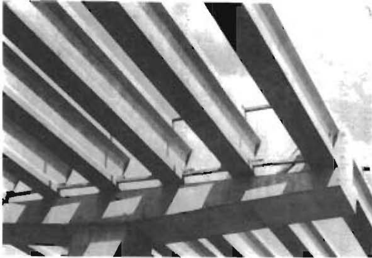
(c) Temporary braces at the end of the span
