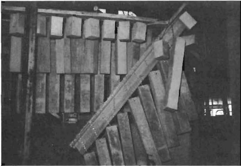
Fig. 5.50 Bridge 1 after failure.
