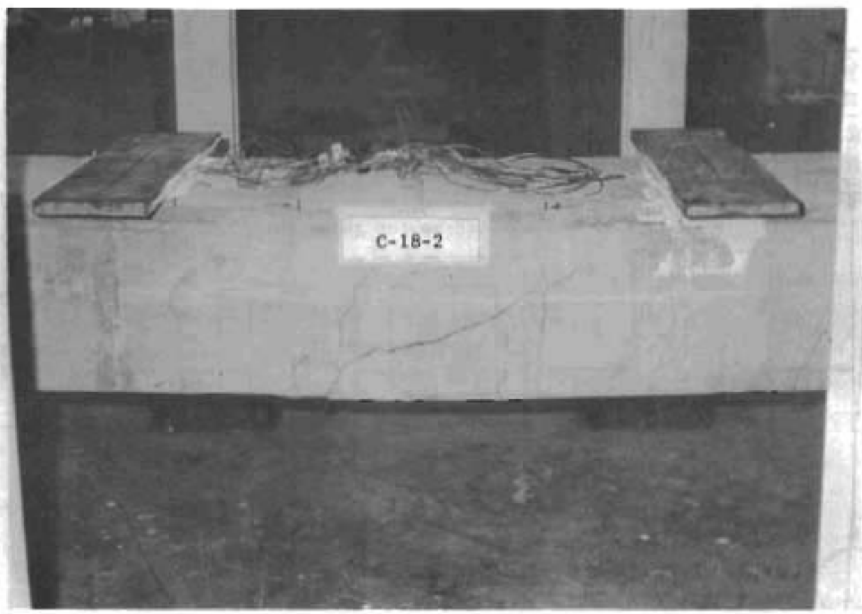
Fig. 2.5. Specimen C-18-2 after failure
