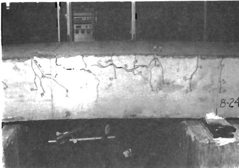
Fig. 3.5. Side view of 8-24-4/2/2-6/6 after failure
