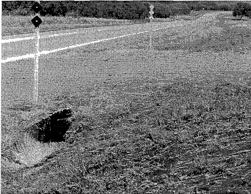
Figure 6.8: Steep slopes on the side of a driveway
