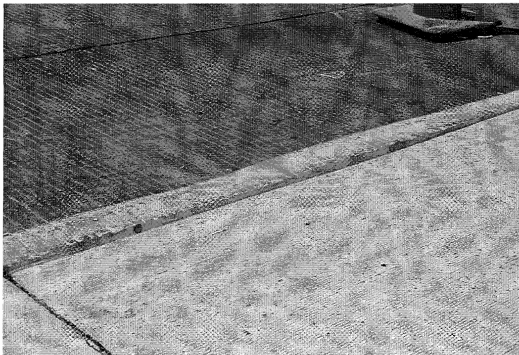
Figure B.2: Surface profile before and after grinding. Note U.S. pennies (1.9 cm diameter at deepest cuts).
