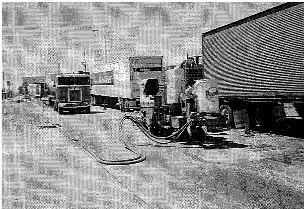
Figure B.1: Pavement surface recondition for WIM installation.
