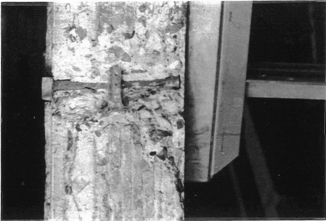
Figure 50 Excavation of study in roadway section
