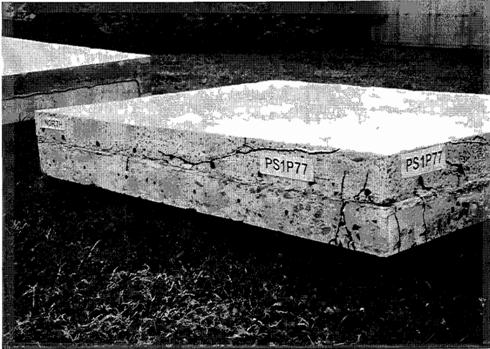
Figure 8.7: Saw cut face (longitudinal section) of precast prestressed panel pulsating fatigue test Specimen PS1P77.
