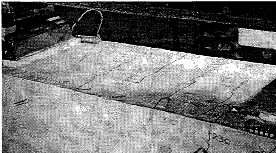
Figure 3.5 Crack Distribution at the Top of Pier A1-1 After Failure
