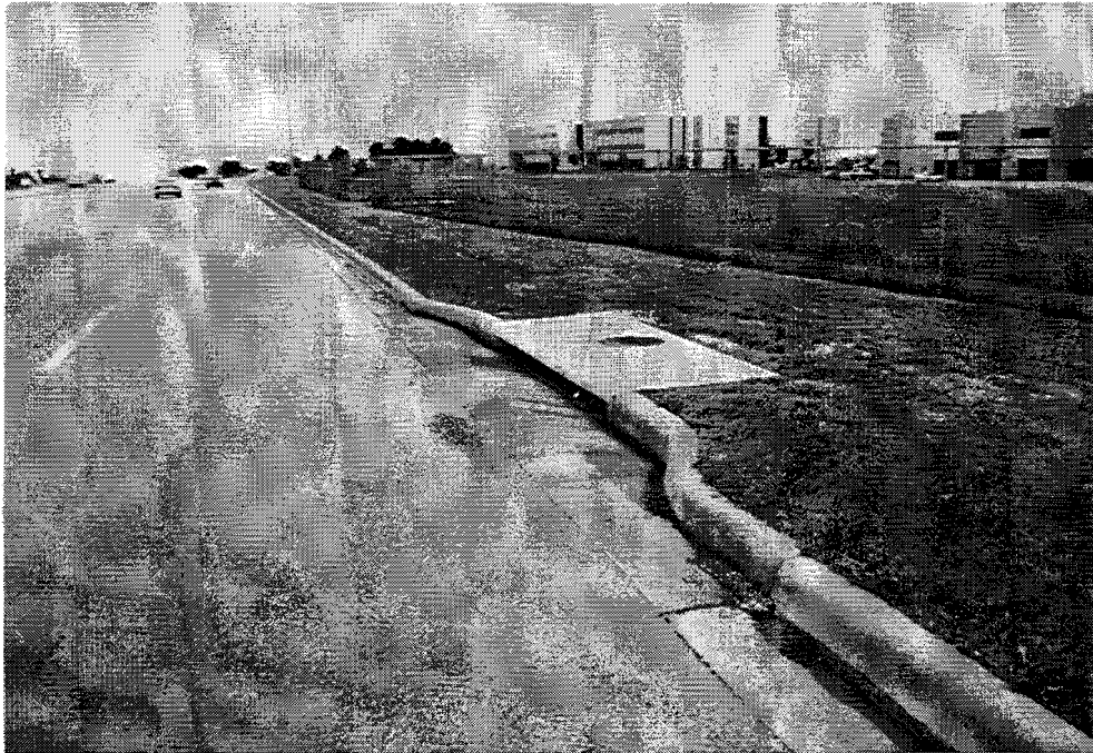
Figure C.1 Recessed curb inlet
