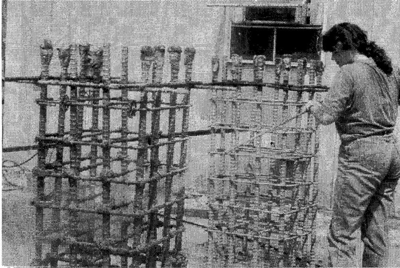
*Figure 2. 10 Washing column cages after vibration*
