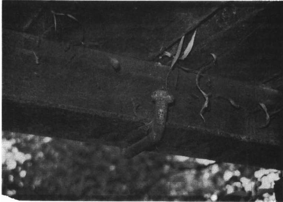
Figure 5.3 Typical J-Bolt Connection at Exterior Stringer
