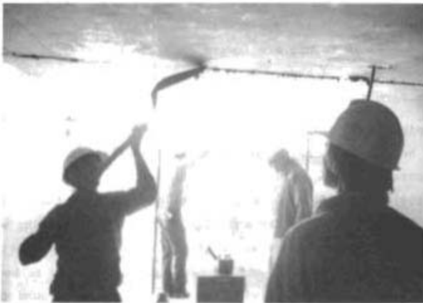
(b) Removal of excess after stressing
