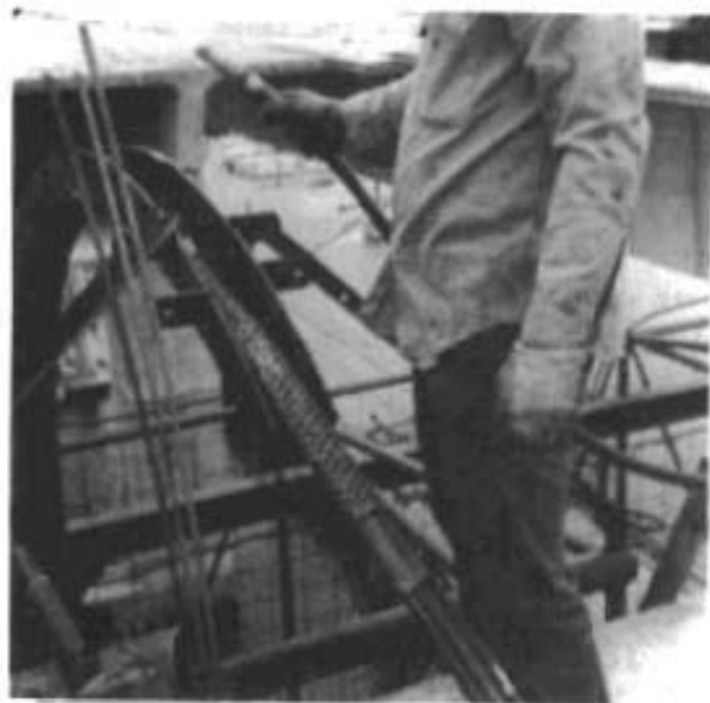
(a) Strand being sprayed with lubricant
