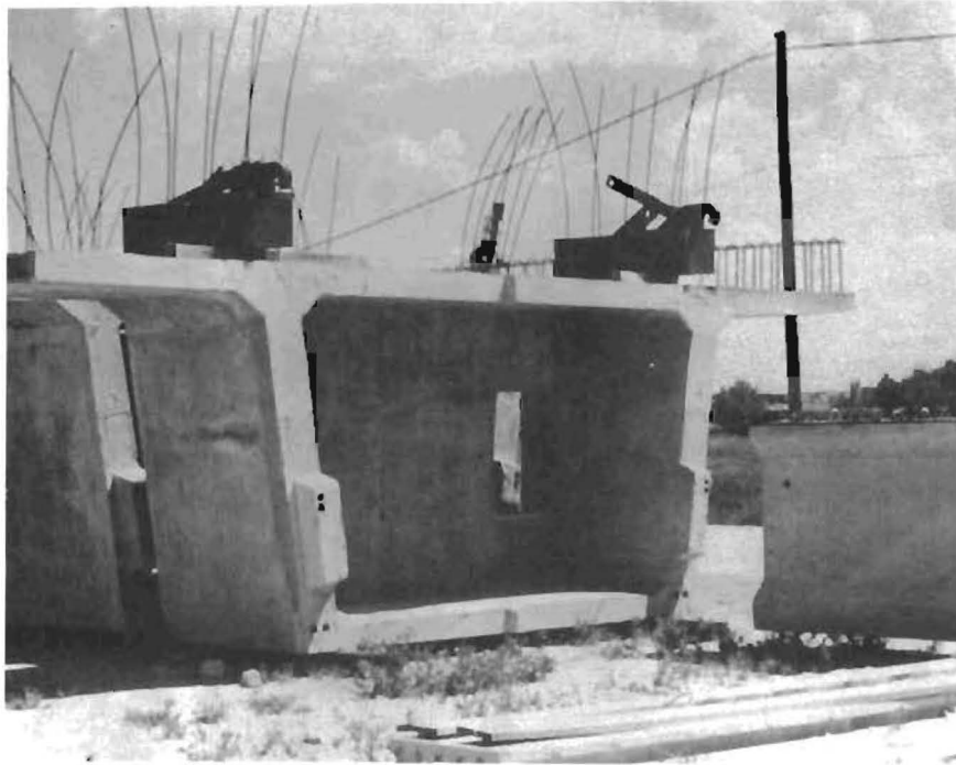
(a) Lifting beam in place
