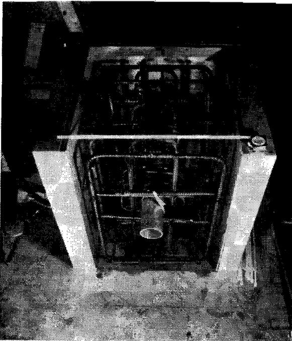
Figure 3.3 Deviator Block Formwork.
