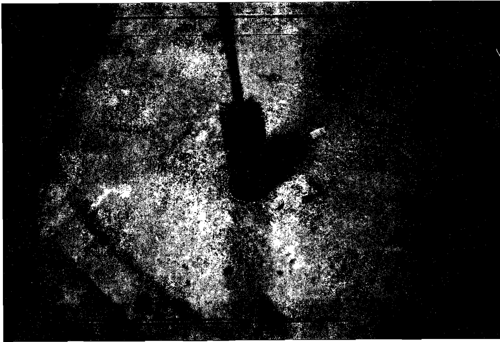
Figure 4.5 Cleaning holes with bottle brush.
