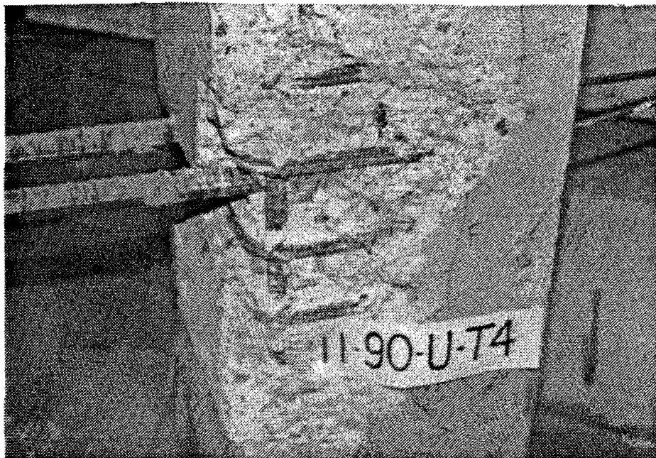
Figure 8.18 Joint region of the #11 uncoated hooked bar specimen of the fifth series, #3 at 4 in., f'_c = 4225 psi.
