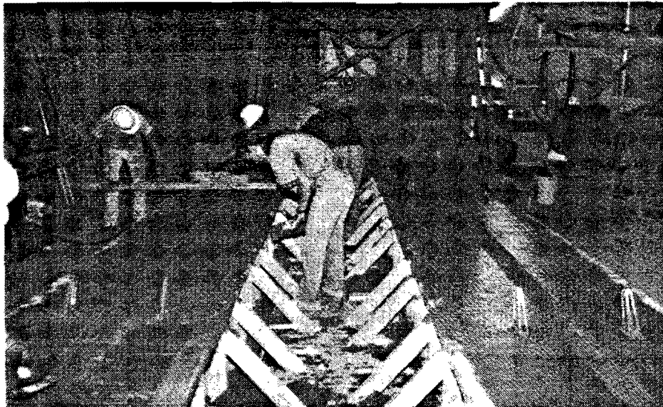
(b) Screeding and trowelling the beam surface
