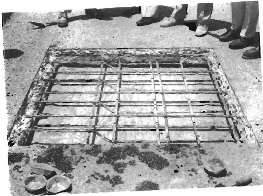
Fig. 5.4. Bridge on U.S. 80 After Placement of Form.
