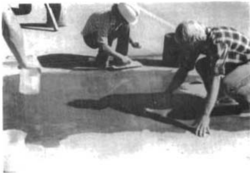
Fig. 5.2. Finishing MoPac Boulevard Repair.
