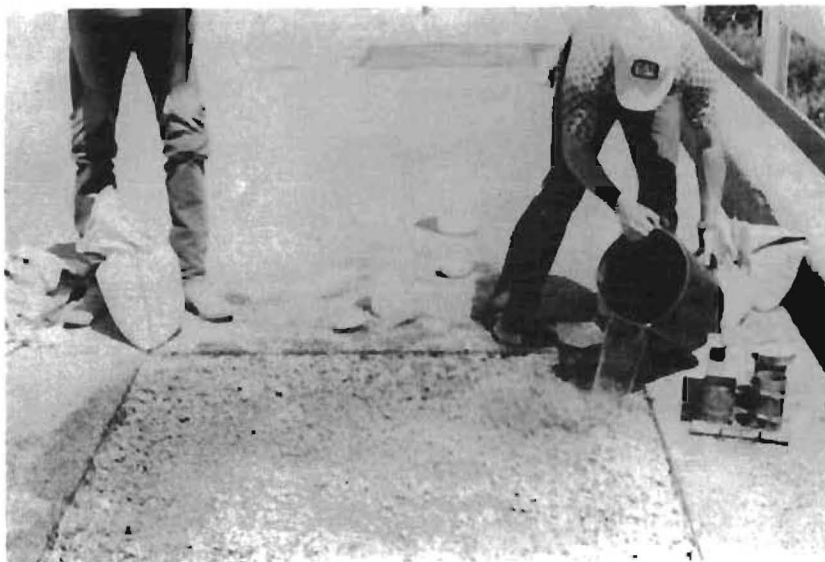
Fig. 5.5. Monomer Application.
