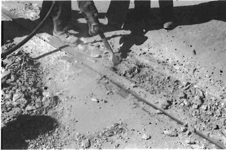
Fig. 5.12. Removal of Deteriorated Concrete.
