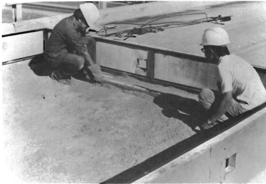
Fig. 4.3 Screeding Sand to Thickness of 0.375 in.
