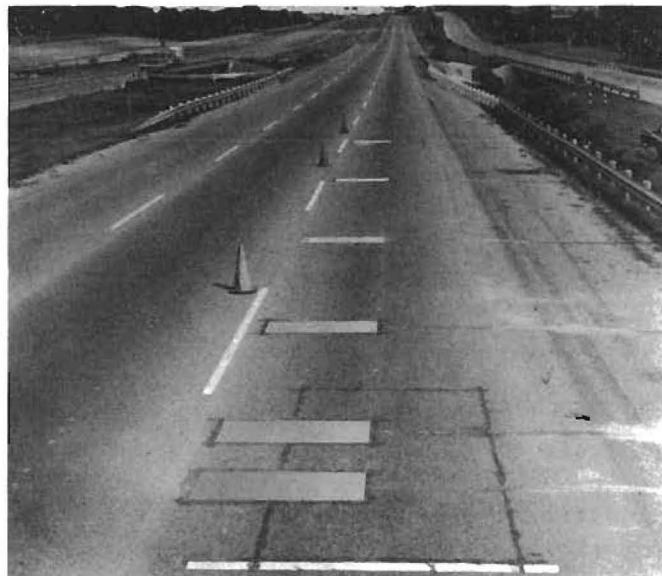
Fig 36. View of field installation.
