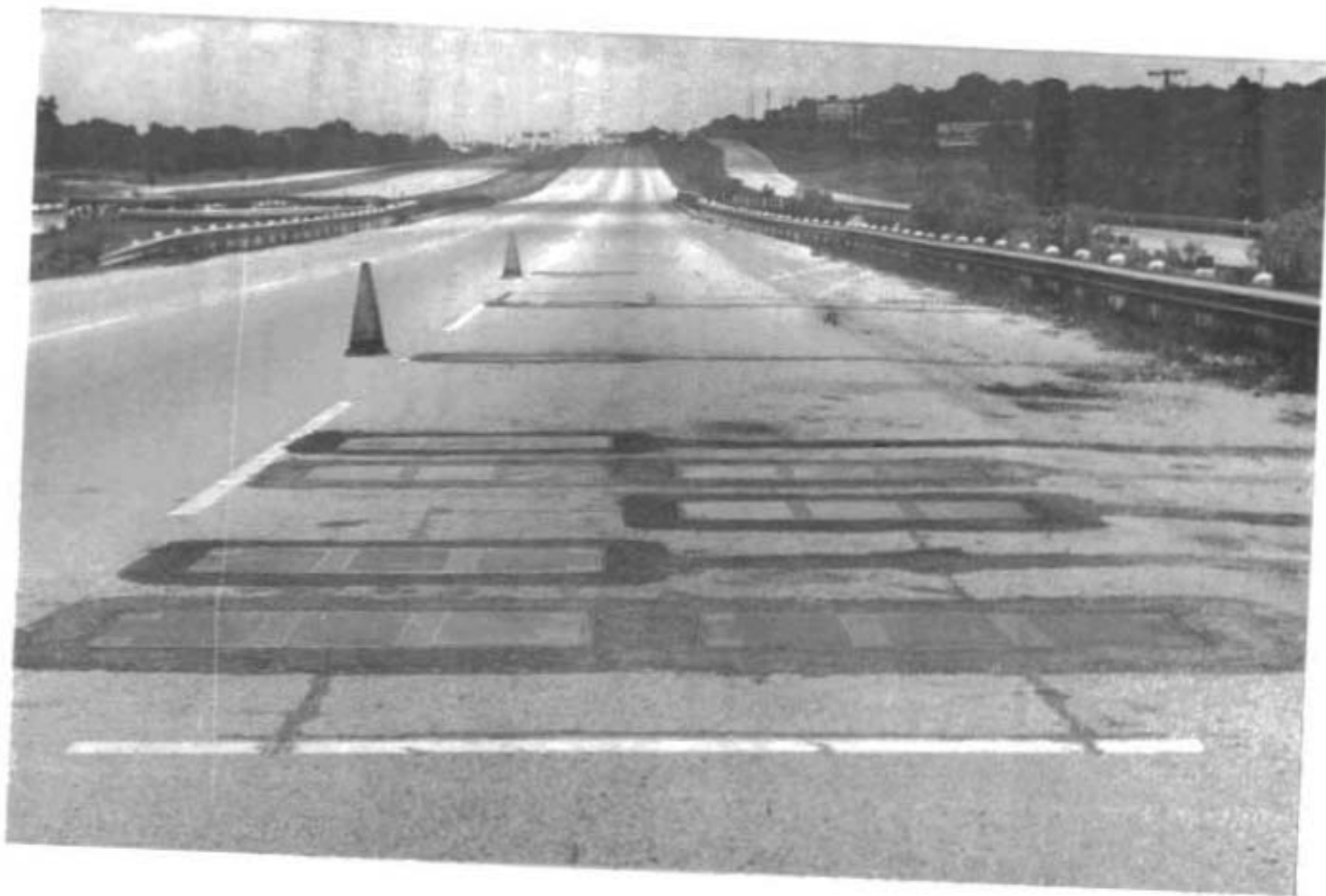
Fig 38. Driver view of field installation.
