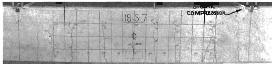
(c) Side of beam. Shear compression failure from loading arm.
