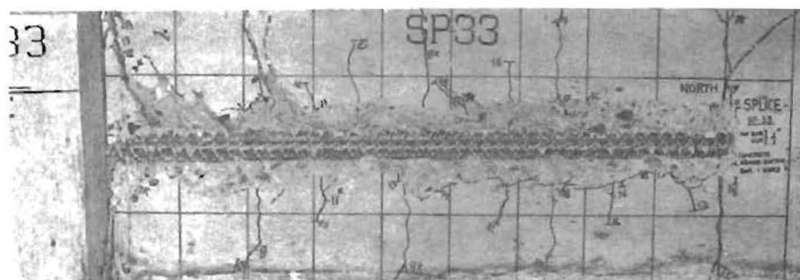
(b) The failed surface, V-type.
