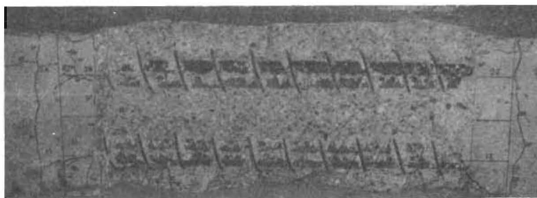
(a) Failure #18 splice with 3/8 in. spiral at 6 in., L_s = 60 in.
