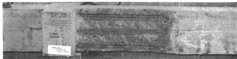
(b) Failure surface.
