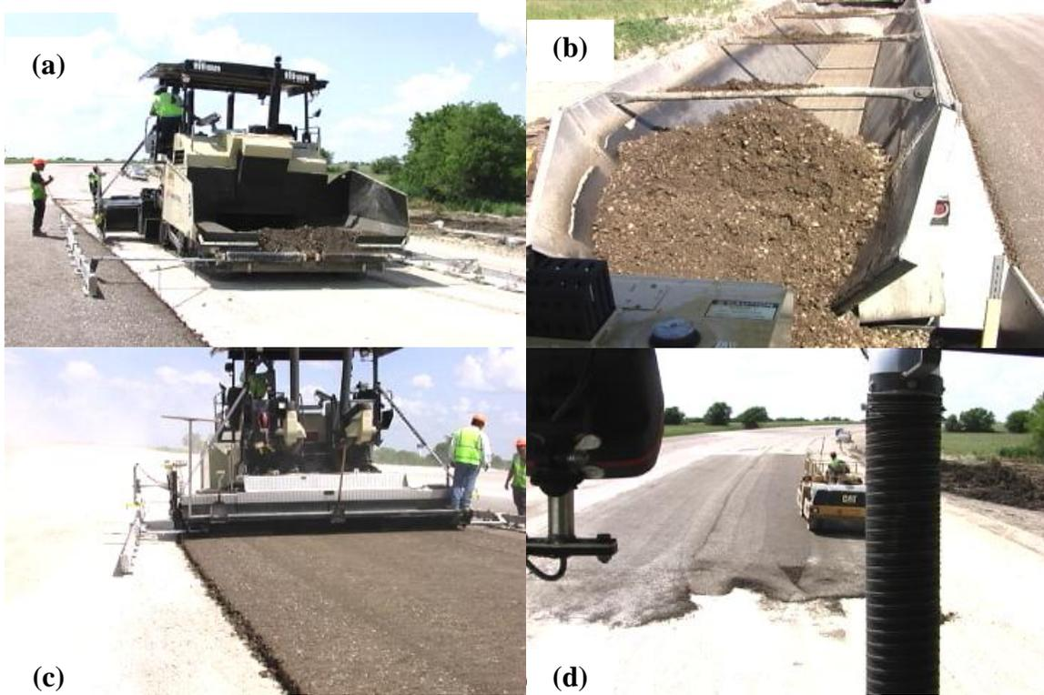
**Figure 11** Base Lay-down Machine (a) Hopper and its Conveyor (b) Unloading Base Material Transported from Pugmill to Hopper (c) Lay-down of Emulsified Asphalt Base in Progress (d) Rolling of Laid-Down Base
