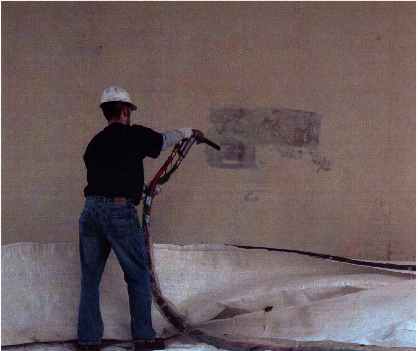
Initial blasting with dry ice. Note lack of dust.
