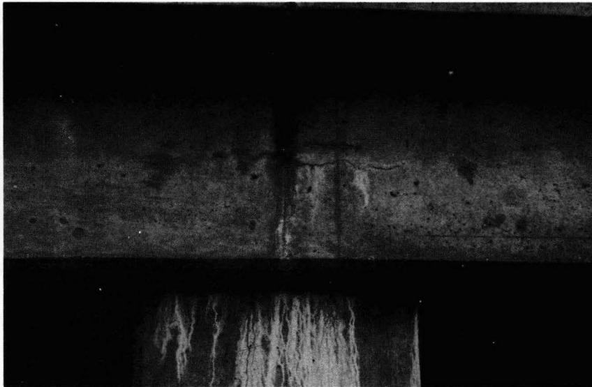
(b) Continuous Slab Structure Note horizontal cracks at joint
