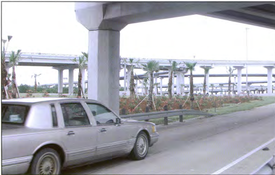
Innovative construction sequencing allowed lanes on Beltway 8 Tollway (in Houston) to open 45 days earlier than scheduled, and the project to be completed three months ahead of schedule.
