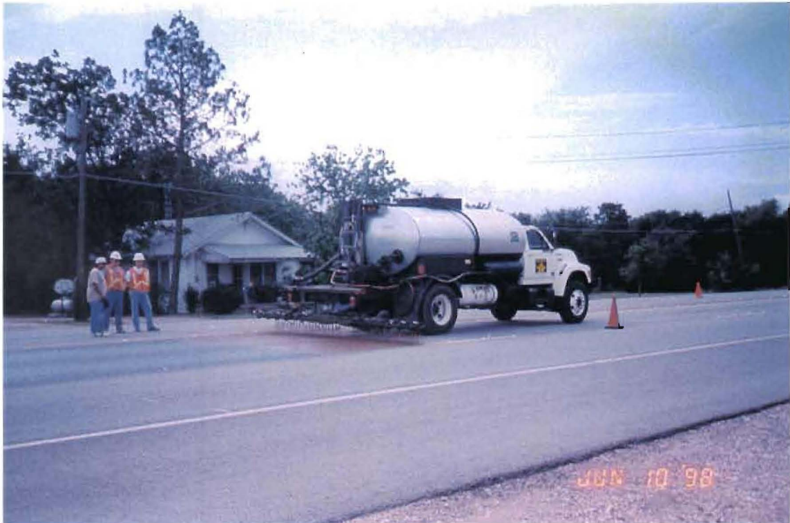
Application of Reclamite for Phase II Test Section.
