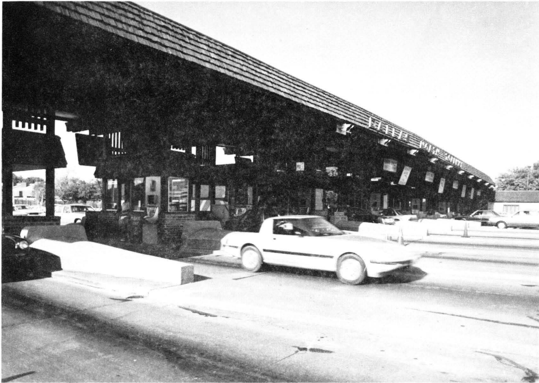
Dallas North Tollway Barrier Plaza No. 1
