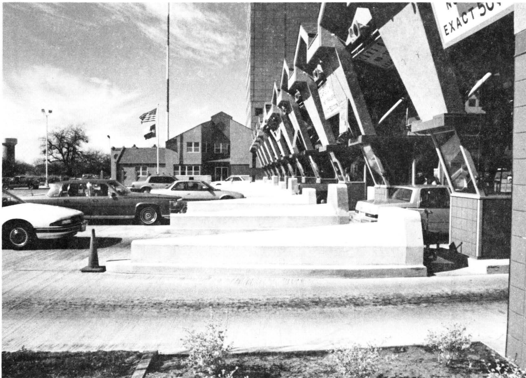
Dallas North Tollway Barrier Plaza No. 2
