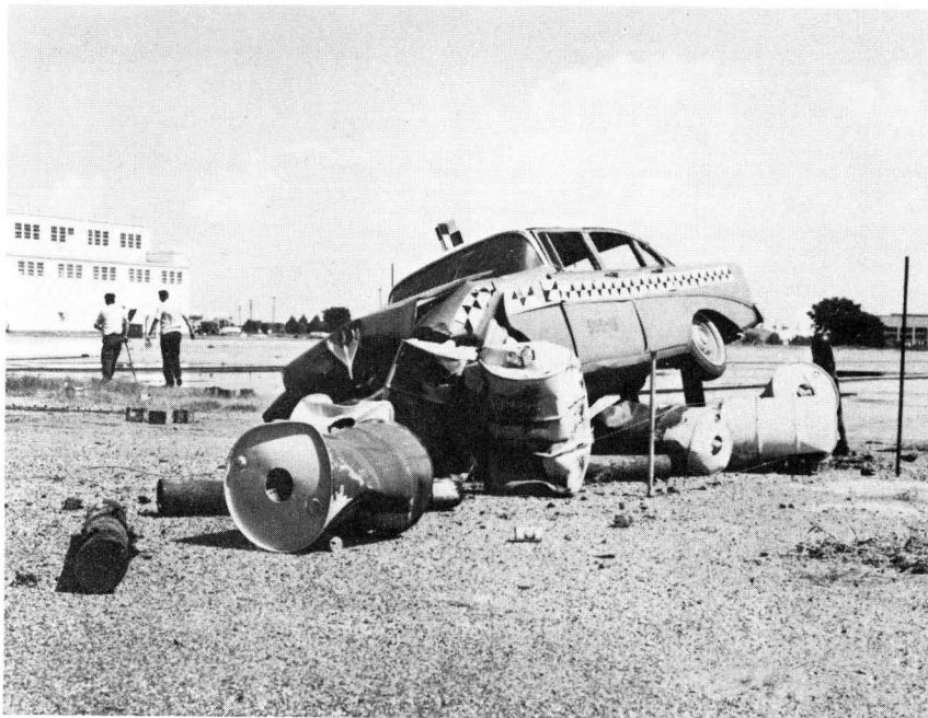
FIGURE 4. BARRIER AND VEHICLE AFTER TEST 505-1B.
