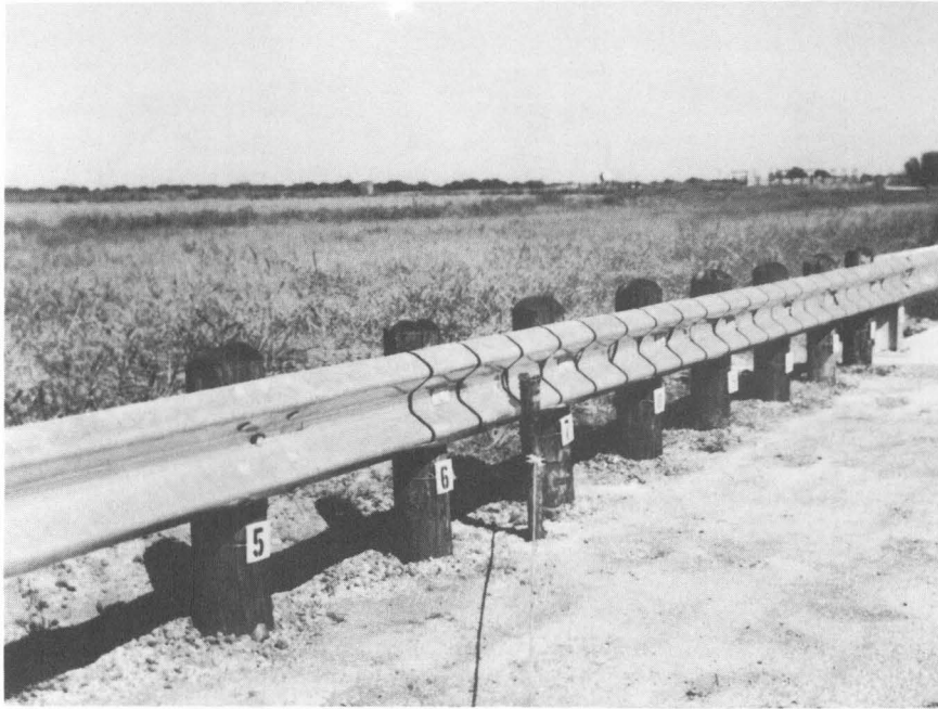
Figure 19, Guardrail Installation Before Test T1-C.
