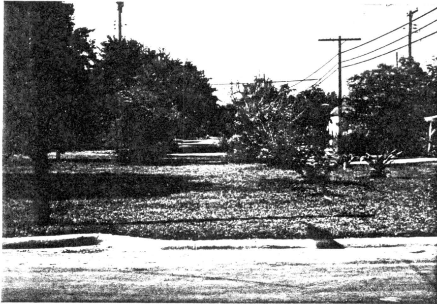
Figure 4-10 Elimination Of Intersection Of Local Street With A Major Street Bordering A Neighborhood In Edinburg, Texas
