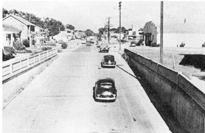
The inadequacies of old traffic arteries are shown in this photograph of Polk Avenue taken from H.B.&T.R.R. underpass. Note narrow roadway and heavy commercialization of abutting property.
