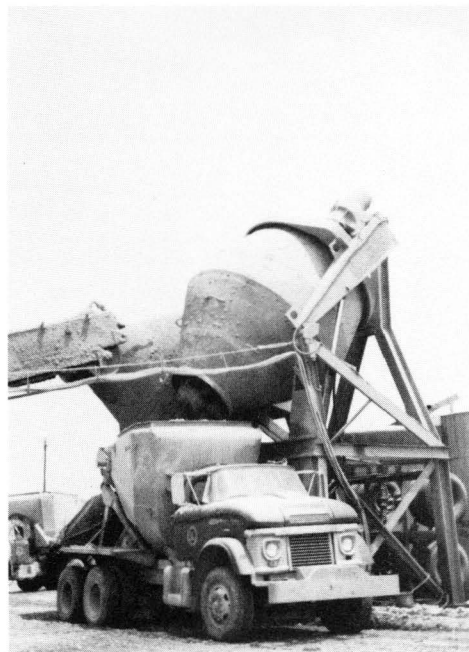
FIGURE 25. 9-YARD MIXER DUMPING INTO "AGITOR" WET BATCH TRUCK AT CENTRAL MIX PLANT.
