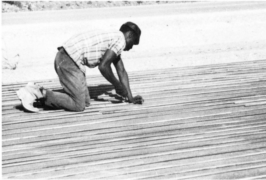
FIGURE 44. LONGITUDINAL STEEL BEING TIED AT SPLICES; NOTE STAGGERED SPLICE PATTERN.
