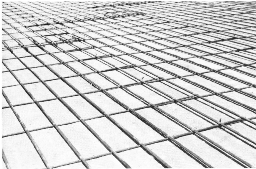
FIGURE 66. TIED WELDED WIRE FABRIC REINFORCEMENT READY FOR FINAL POSITIONING ON CHAIRS.
