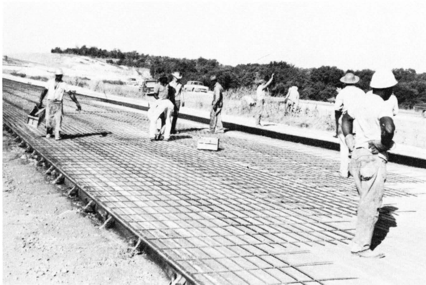
FIGURE 64. TYING WELDED WIRE FABRIC AT SPLICES.
