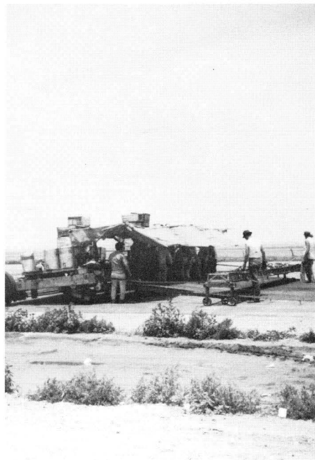
FIGURE 53. SIDE VIEW OF EQUIPMENT FOR FABRICATING REINFORCING STEEL MAT FROM DEFORMED STEEL BARS; TRANSVERSE STEEL IS BEING TIED TO LONGITUDINAL STEEL BENEATH CANOPY; TRAILER CARRIES PRESSED STEEL CHAIRS USED TO SUPPORT MAT.
