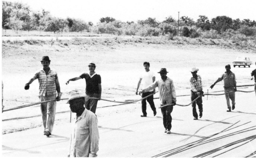
FIGURE 40. INITIAL STAGE OF PLACING LONGITUDINAL REINFORCEMENT COMPOSED OF DEFORMED STEEL BARS.
