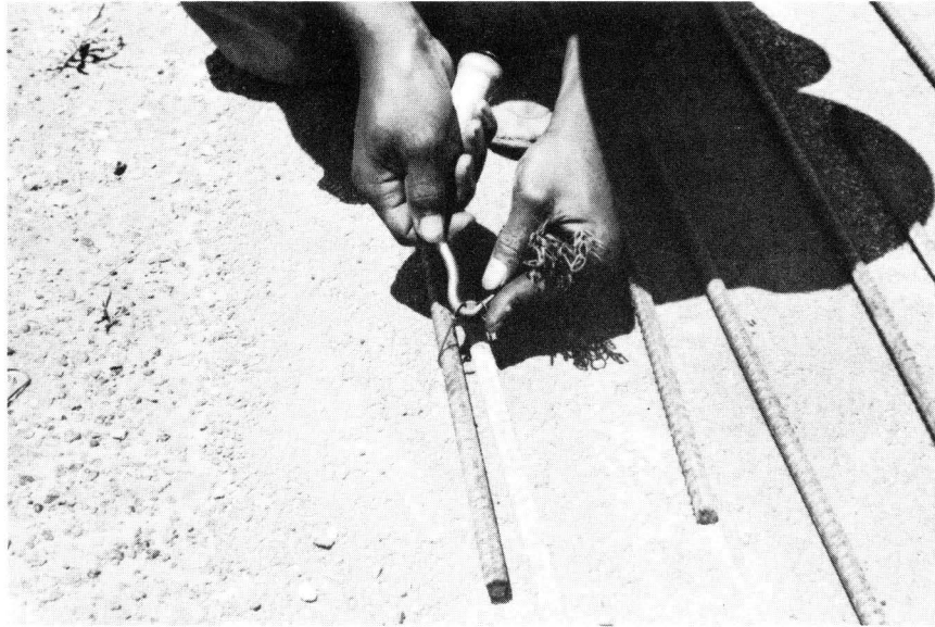
FIGURE 42. INITIAL STAGE OF TYING OPERATION AT SPLICE IN LONGITUDINAL STEEL.
