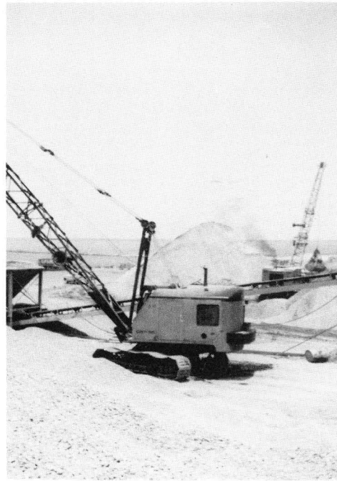
FIGURE 22. STOCKPILE SAND (BACKGROUND) AND HARD SILICEOUS. AGGREGATE ADJACENT TO HIGH-CAPACITY CENTRAL MIX CONCRETE PLANT. BULLDOZERS MOVE MATERIALS TO CRANES WHICH FEED CONVEYOR TO BATCHING PLANT.
