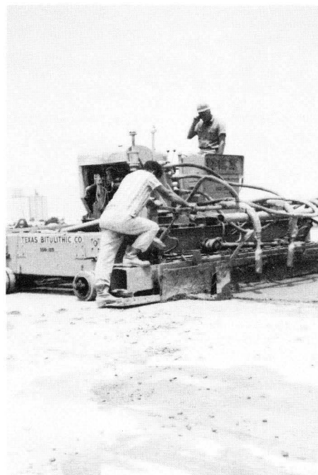
FIGURE 37. PAVER USED IN CRCP PROJECT IN TEXAS. MECHANICALLY DRIVEN VIBRATORS CAN BE SEEN AT RIGHT. PREVIOUSLY PAVED 12-FOOT LANE IS IN FOREGROUND.
