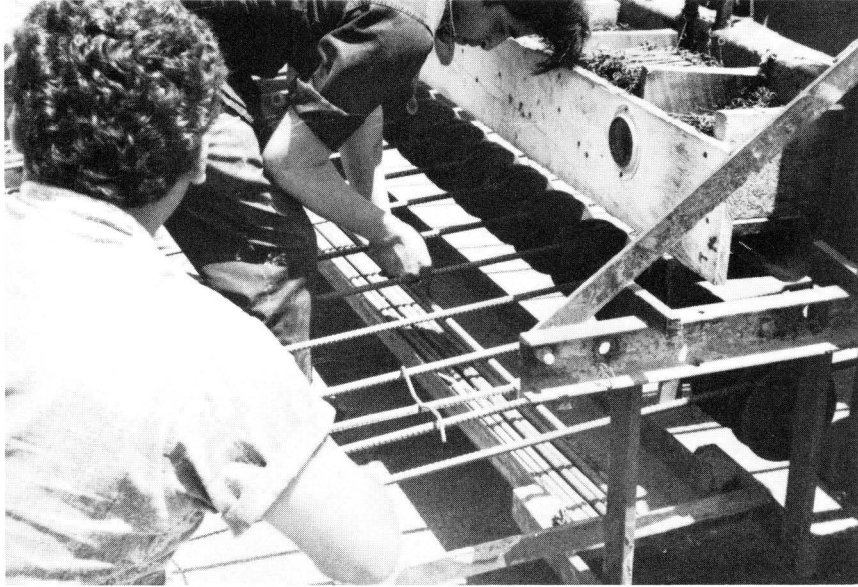
FIGURE 46. TRANSVERSE STEEL BEING TIED TO LONGITUDINAL STEEL.
