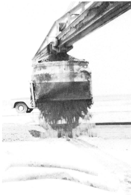
FIGURE 39. CONCRETE BEING PLACED FOR A 12-FOOT LANE BY THE TRAVELING MIXER SHOWN IN FIGURE 38. REINFORCING STEEL IS TIED DEFORMED STEEL BAR; PREVIOUSLY PAVED 12-FOOT LANE IS IN FOREGROUND.
