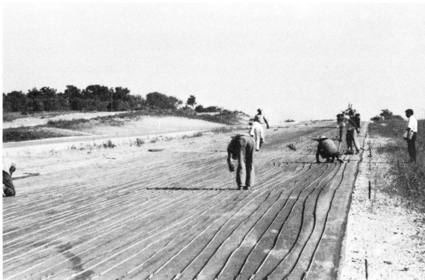
FIGURE 45. CREW TYING AND ALIGNING LONGITUDINAL STEEL.
