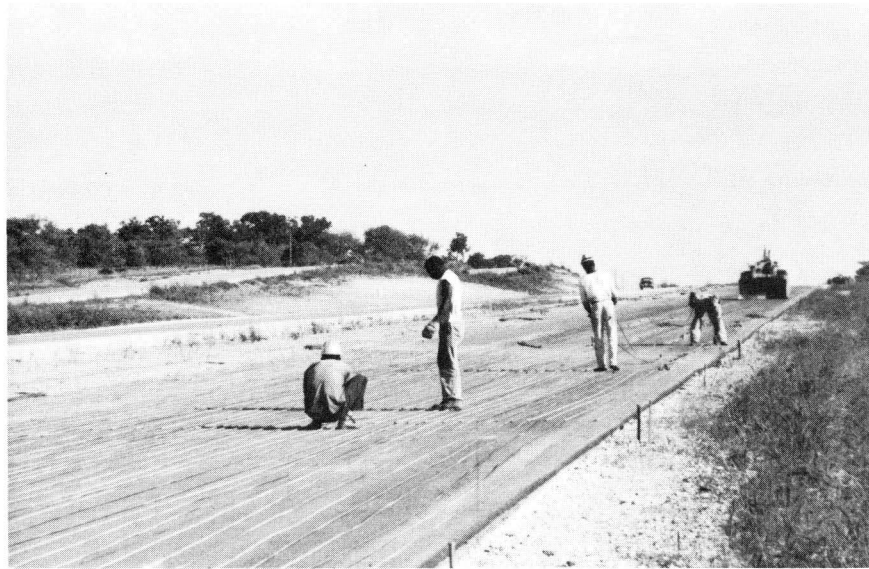
FIGURE 41. INITIAL POSITIONING OF LONGITUDINAL STEEL PREPARATORY TO SPLICING AND TYING.
