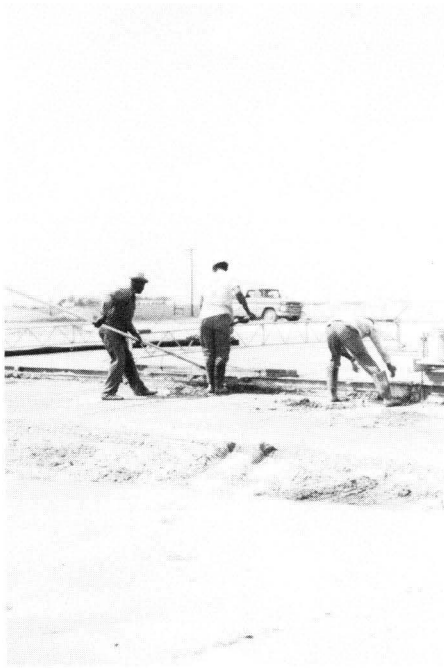
FIGURE 33. PORTION OF CONCRETE SURFACE FINISHING OPERATIONS FOLLOWING SLIP-FORM PAVER.
