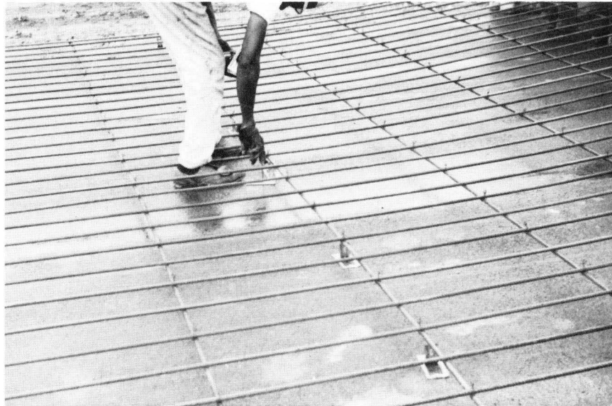
FIGURE 51. SPACING OF STEEL CHAIRS SUPPORTING TIED DEFORMED STEEL BAR MAT.
