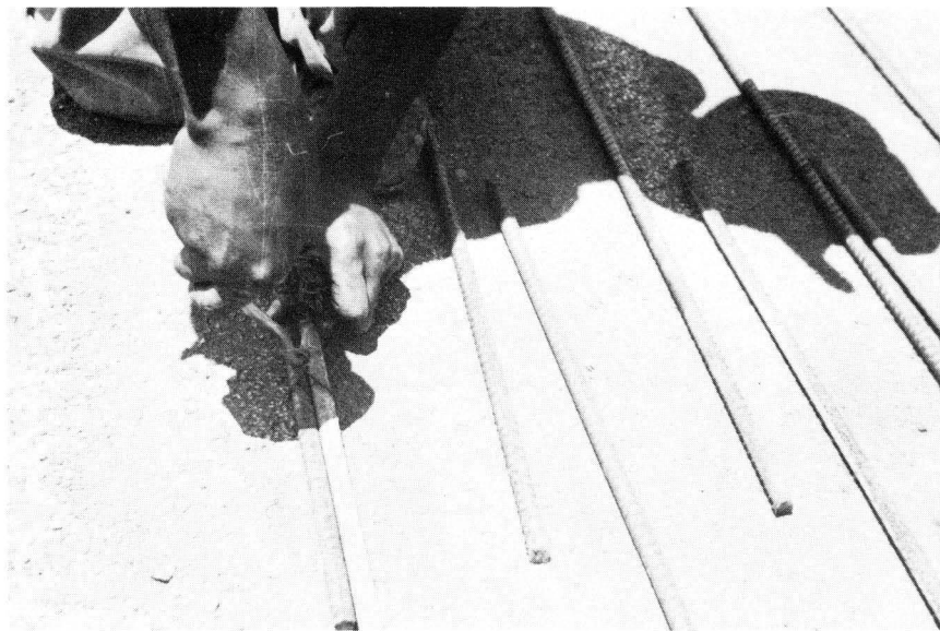
FIGURE 43. FINAL TWIST BEING APPLIED TO TYING WIRE AT SPLICE.
