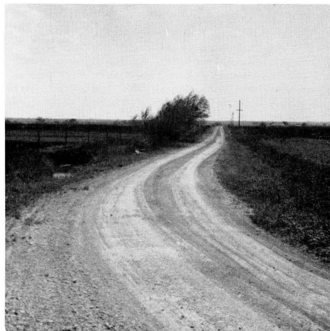
A county-maintained gravel road.
