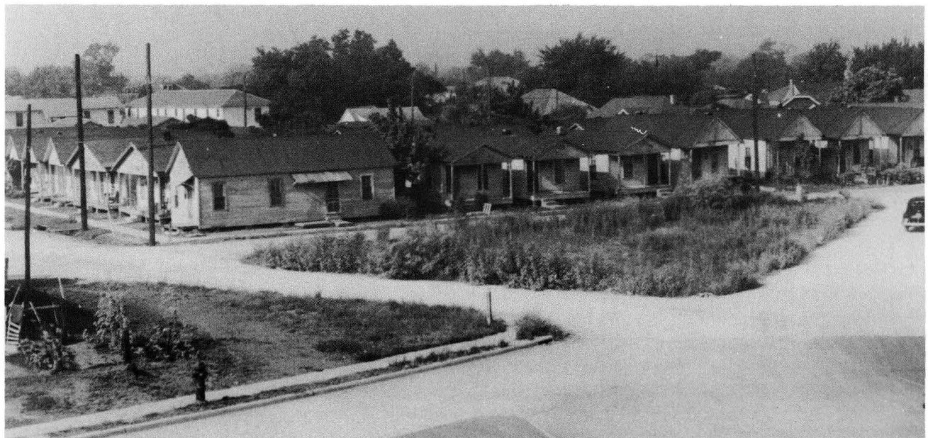
PLATE 10 Across Freeway From Building - Plate 9
