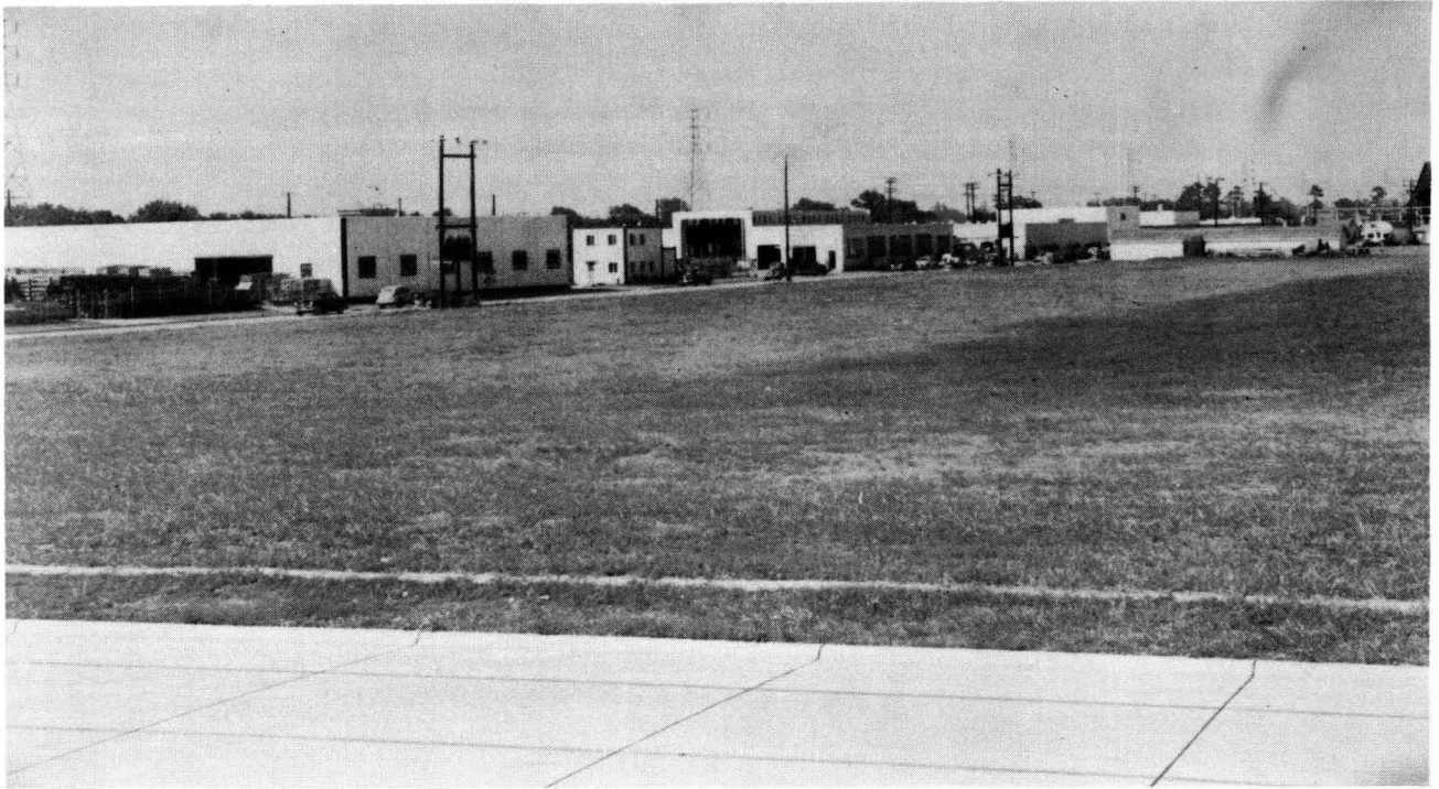
PLATE 15-A New Warehouses North of Freeway - Section 3, Group 1
