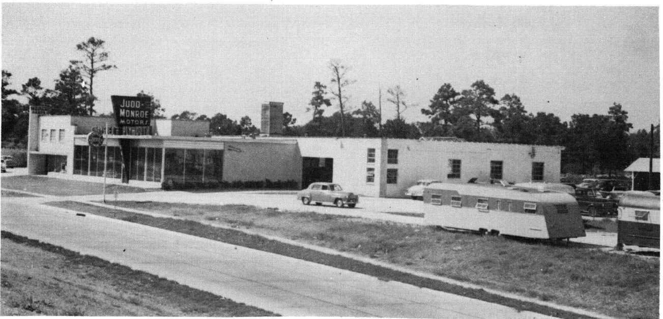
PLATE 17-B Both of Above Views Show New Buildings - Section 4, Group 1
