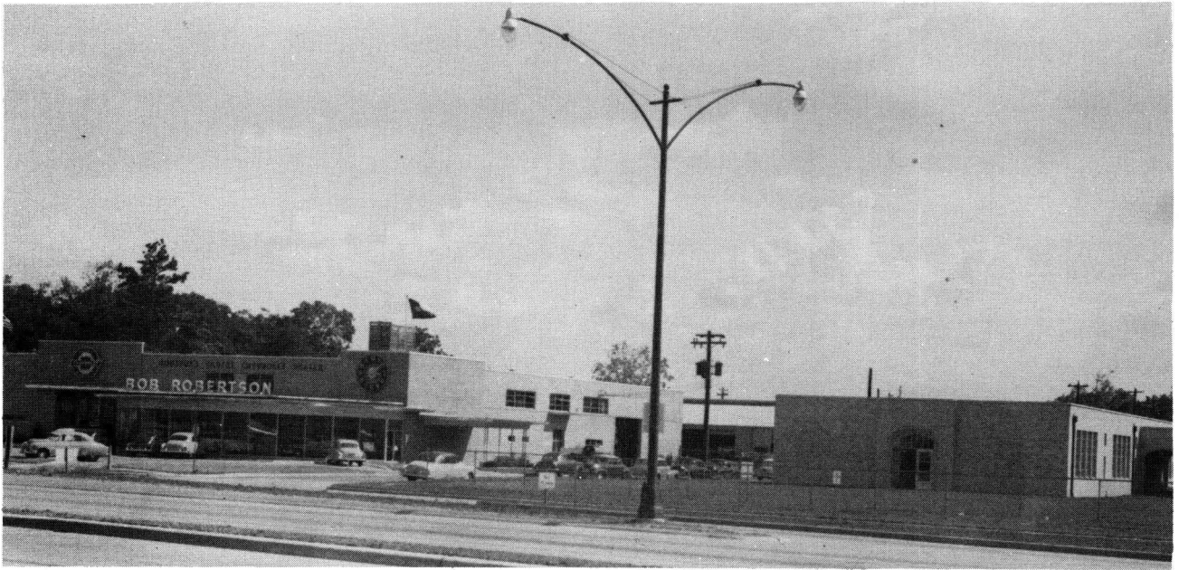
PLATE 17-A Light Standard is Between Off-Ramp and Frontage Road
