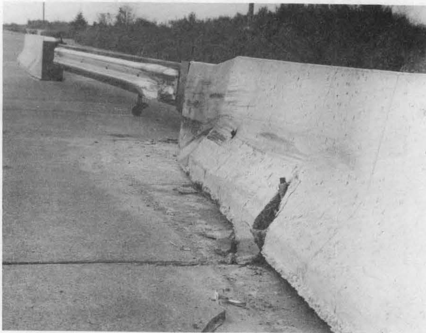
Figure 12. Test Installation Before and After Test 3 (Continued).
