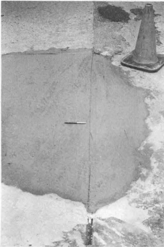
Appearance immediately after placement
