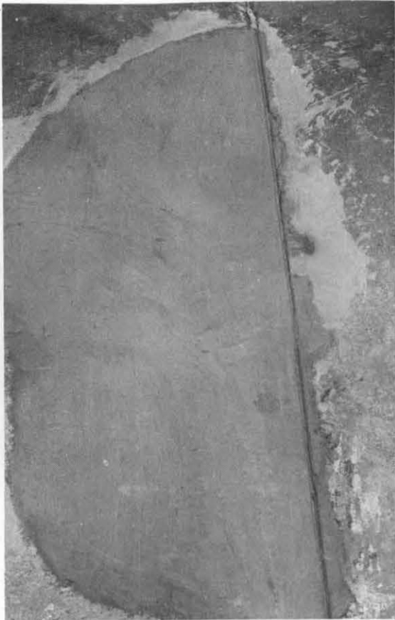
Appearance immediately following placement
