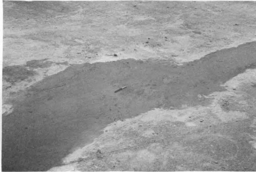
Portion of No. 10 in center lane immediately after placement.
