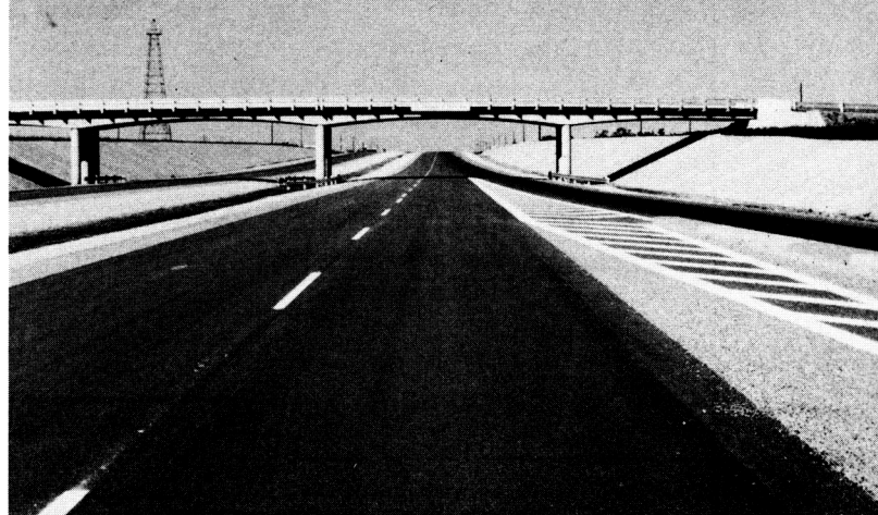
Experimental Approach-End Treatment as Applied to a Freeway Ramp.
