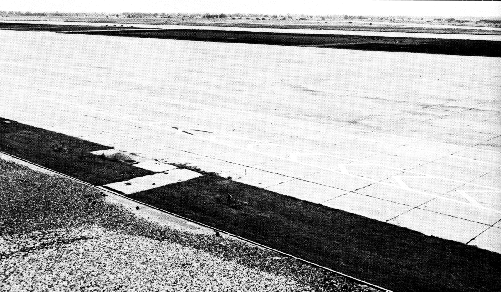
Test Area Showing Layout of Raised Stripe vs. Paint Line.
