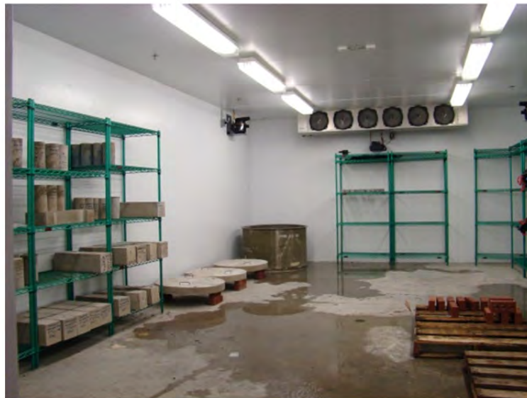
(c) casting and curing space
