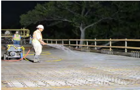
(a) Spraying water on panels
