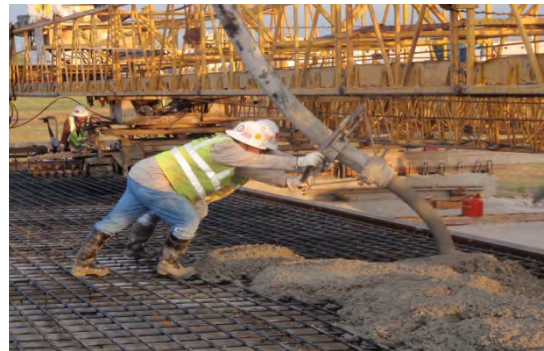
(b) Placing concrete
