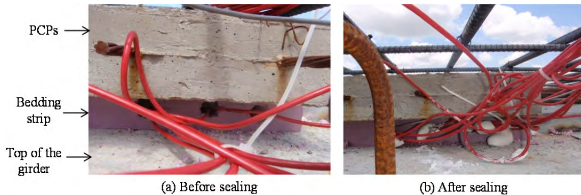
Figure 3-18: Threading wires through holes in bedding strip, Wharton-Weems Overpass
