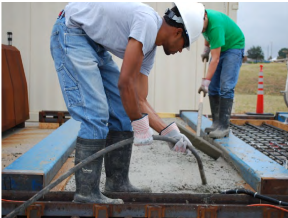
(c) Consolidate with hand-held vibrator
