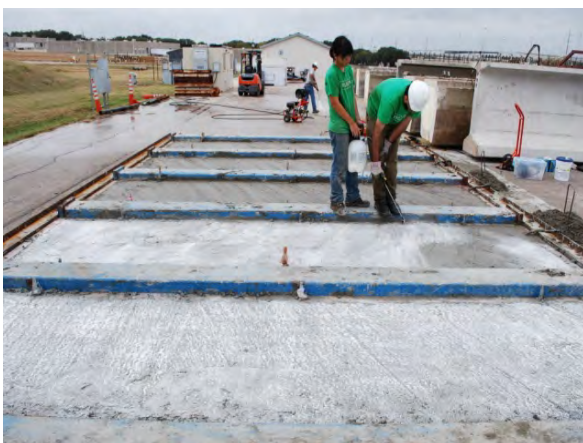
(e) Spray curing compound
