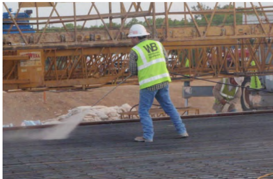
(a) Spraying water on panels
