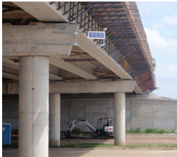
Figure 3-20: Mounting solar panel beside bent cap, Wharton-Weems Overpass
