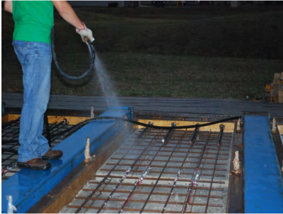
(a) Spray water on panels
