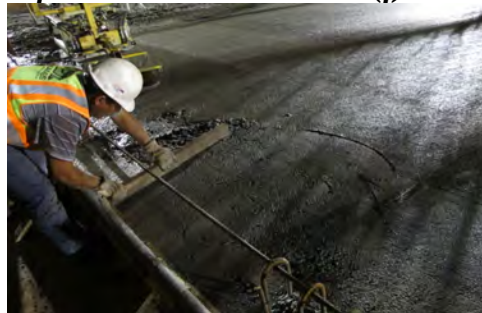
(g) Hand screeding of portion of deck
