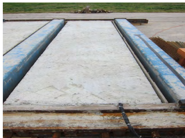
(f) Strip wooden form on one side
