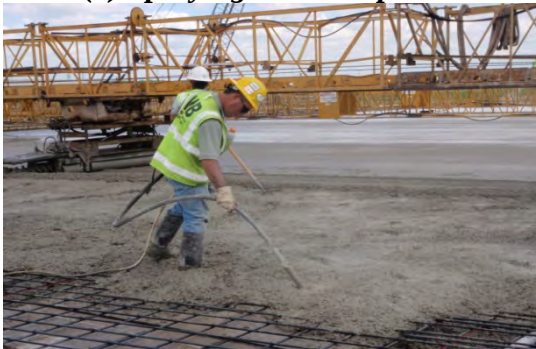
(c) Consolidating concrete
