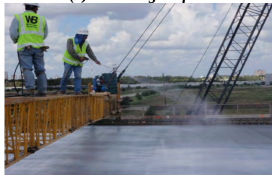
(f) Spraying curing compound on deck surface
