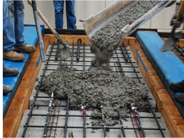
(b) Place concrete
