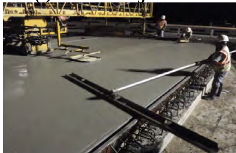
(e) Finishing surface
