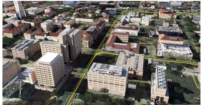
Fig. 9. A 3D overview of the Dean Keeton corridor, spanned by two pedestrian bridges and flanked by buildings on both sides.
