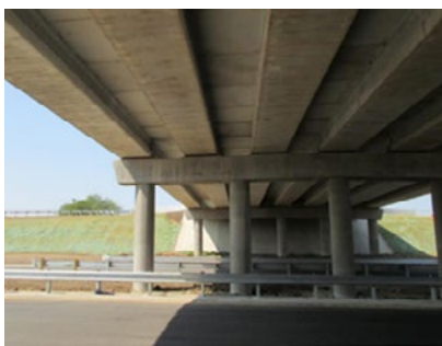
Figure 1 Texas bridge substructure
