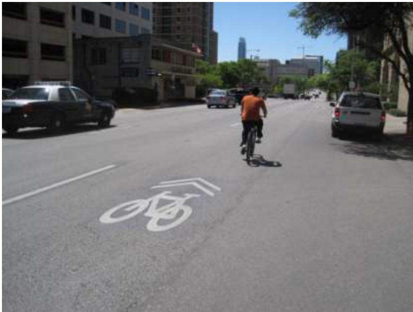
Figure 21. Central placement of sharrow resulted in thriving thermoplastic five months after installation.
