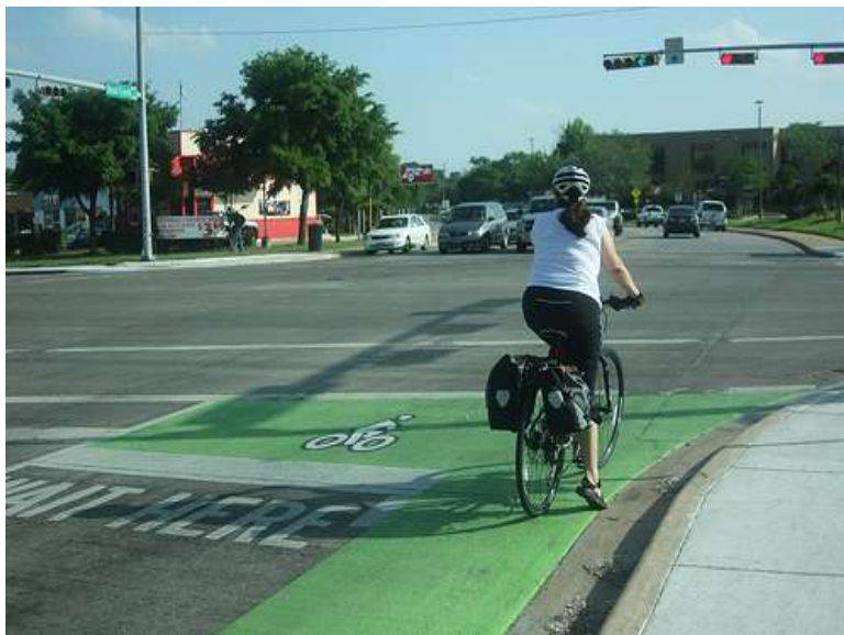
Figure 3. The bicycle box on Shoal Creek Boulevard at Anderson Lane
