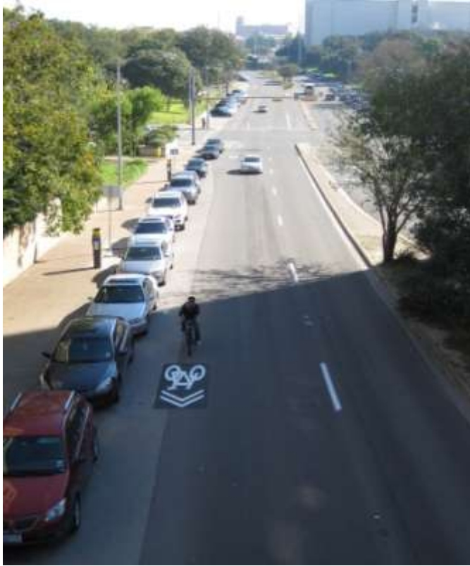
Figure 23. Curb-justified placement of sharrows on west-bound, uphill Dean Keeton Street
