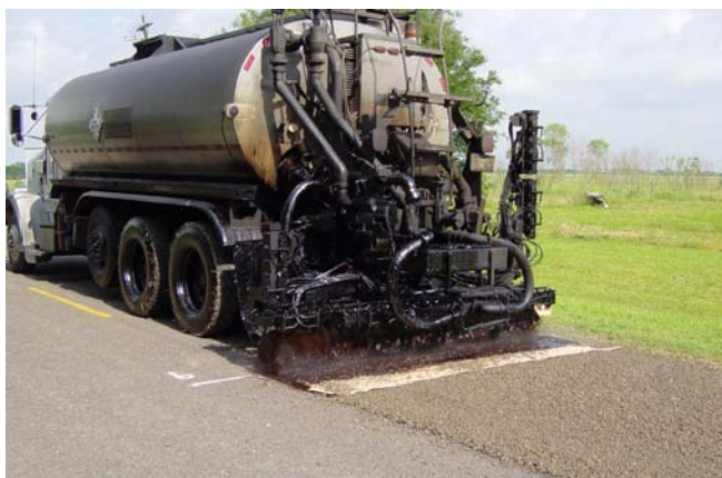
Seal Coat Application
