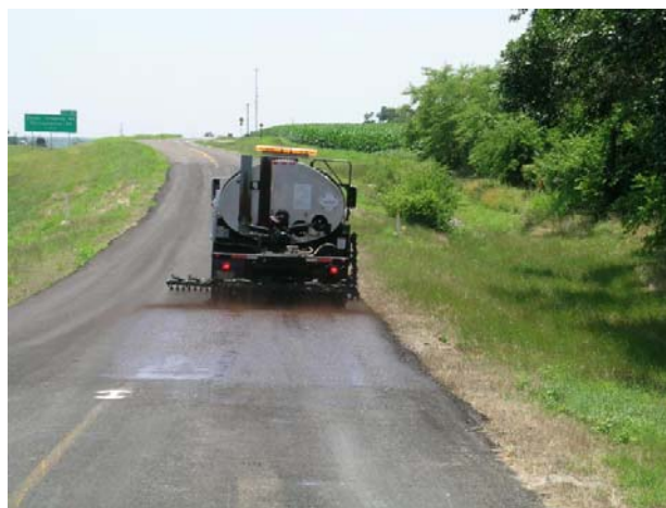
Fresh patches should be fog sealed prior to seal coat application.
