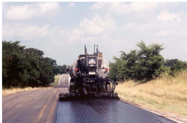
Non-uniform binder application can cause streaking.
