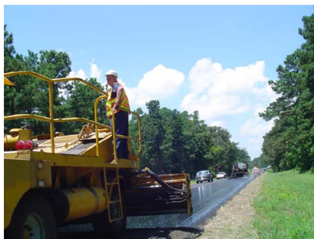
Seal Coat Application
