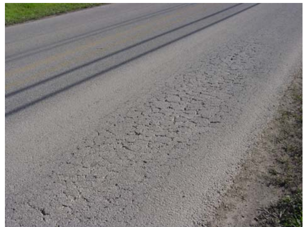
Fatigue Cracking
