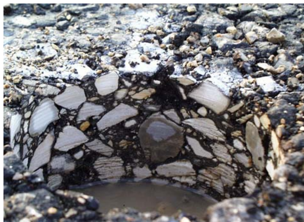
Aggregate breakdown during coring operation
