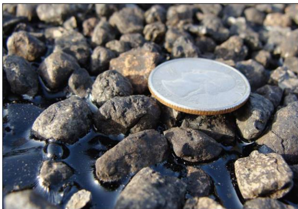
Figure 8. Embedment Slightly Higher than Desired
