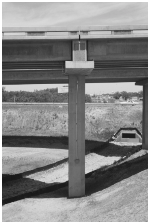
Figure 3.20 - DAS Box with Companion Access Box (San Angelo)
