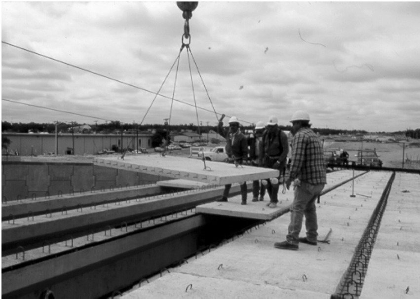
Figure 2.27 - Erection of Precast Panels in the Westbound Bridge
