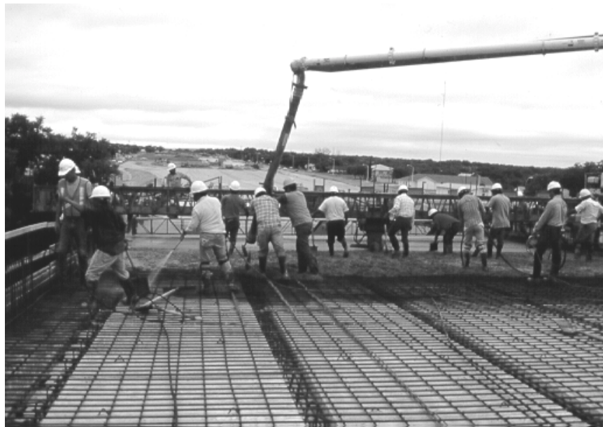
Figure 2.29 - Deck Placement in the Eastbound Bridge
