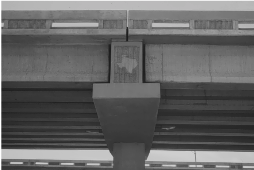
Figure 2.31 - Pier Cap in the North Concho River Overpass
