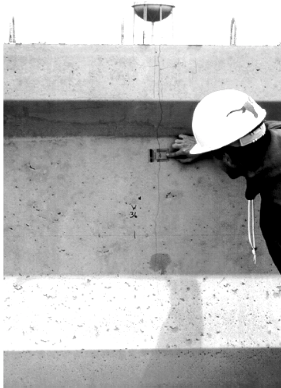
Figure 6.5 - Cracking in a San Angelo HPC Type IV Beam Prior to Release
