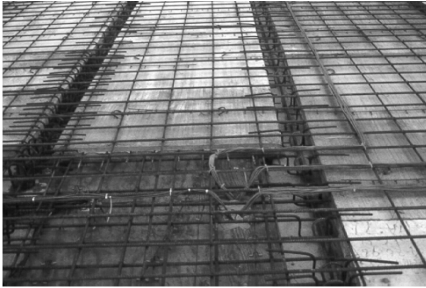
Figure 3.36 - Leadwires Run Through Holes in Deck Formwork Near DAS Box
