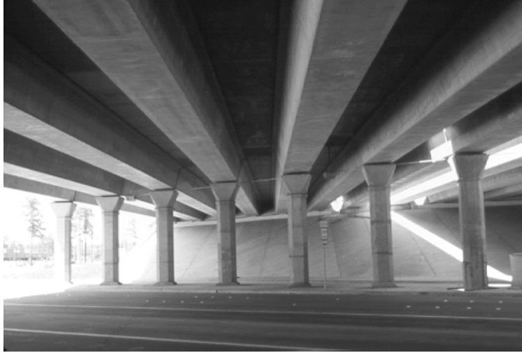
Figure 2.8 - Louetta Road Overpass Substructure
