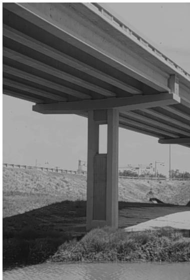
Figure 2.30 - Pier Column in the North Concho River Overpass
