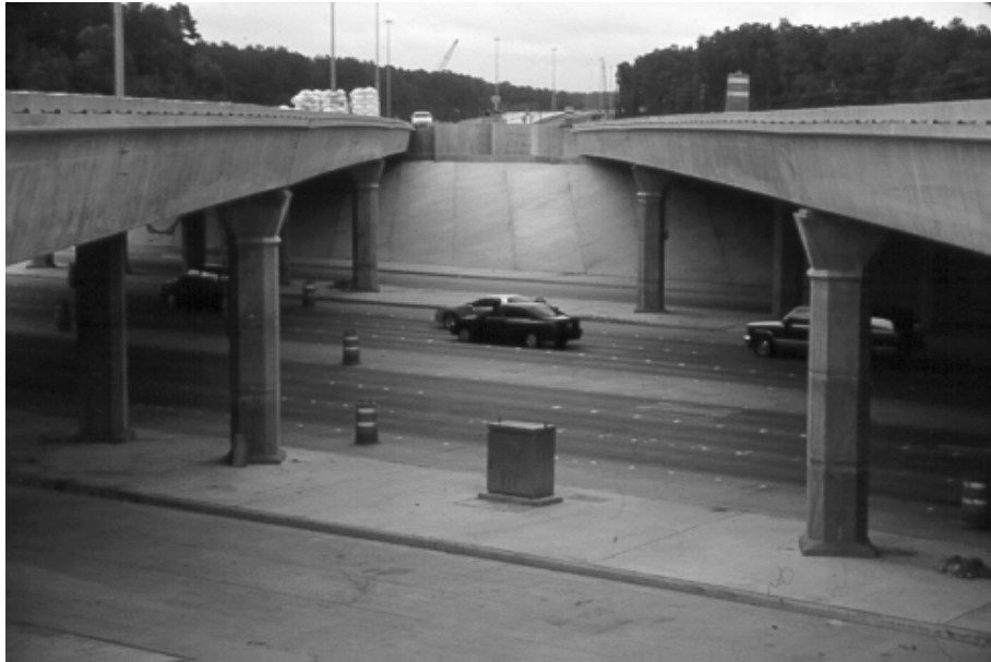
Figure 2.10 - Completed Original Louetta Bridges (Prior to Widening)
