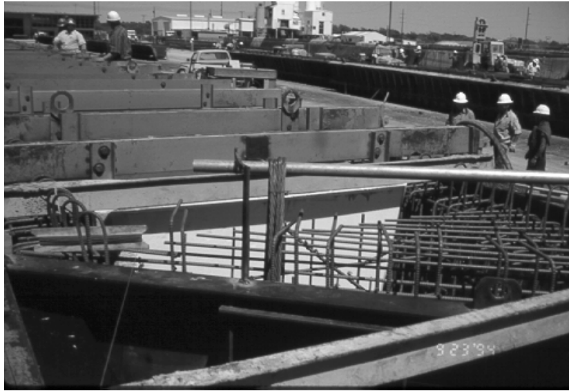
Figure 2.19 - Reinforcement in the Skewed End Block of a Louetta Beam
