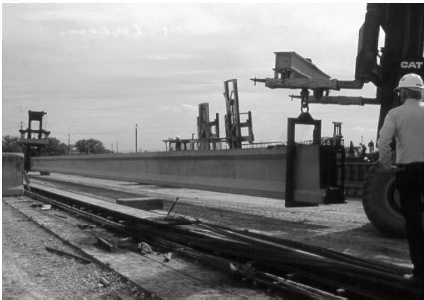
Figure 10.2 - Use of Rigid Lifting Frame for Handling of San Angelo Eastbound HPC Type IV Beams at Prestressing Plant
