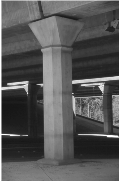
Figure 2.9 - Louetta Road Overpass Substructure
