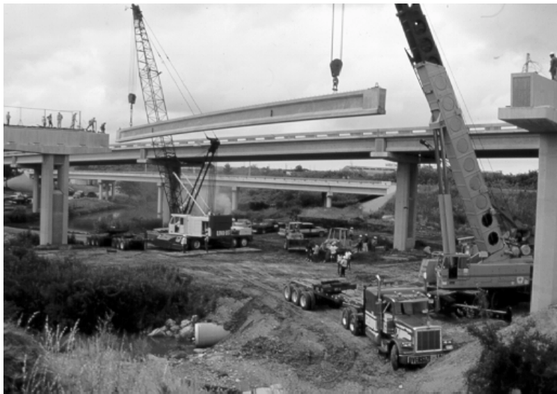
Figure 10.4 - Erection of San Angelo Eastbound HPC Type IV Beams at Jobsite
