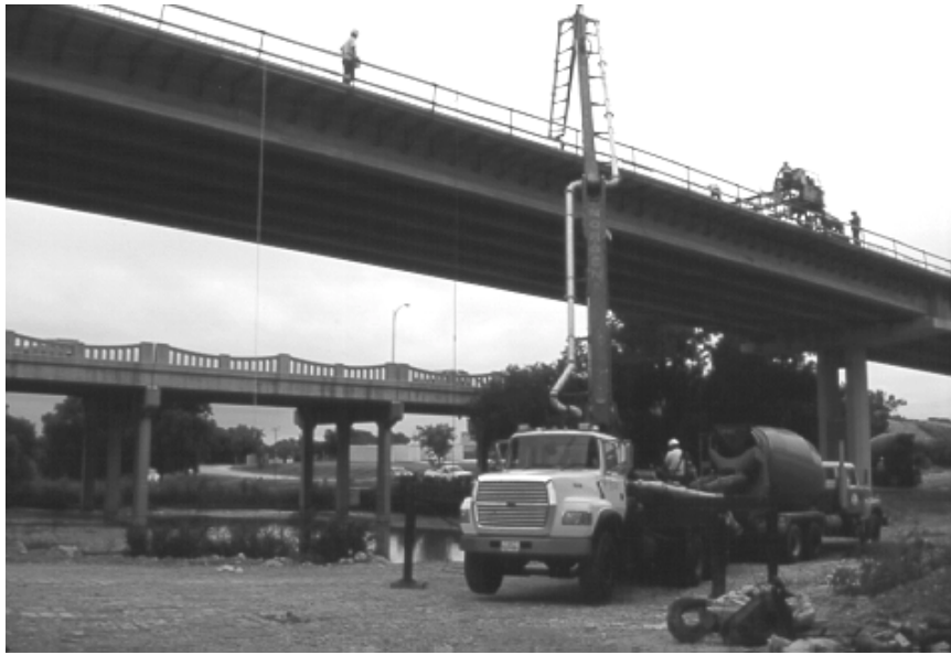
Figure 2.28 - Pumping of Concrete During Deck Pour in the Eastbound Bridge
