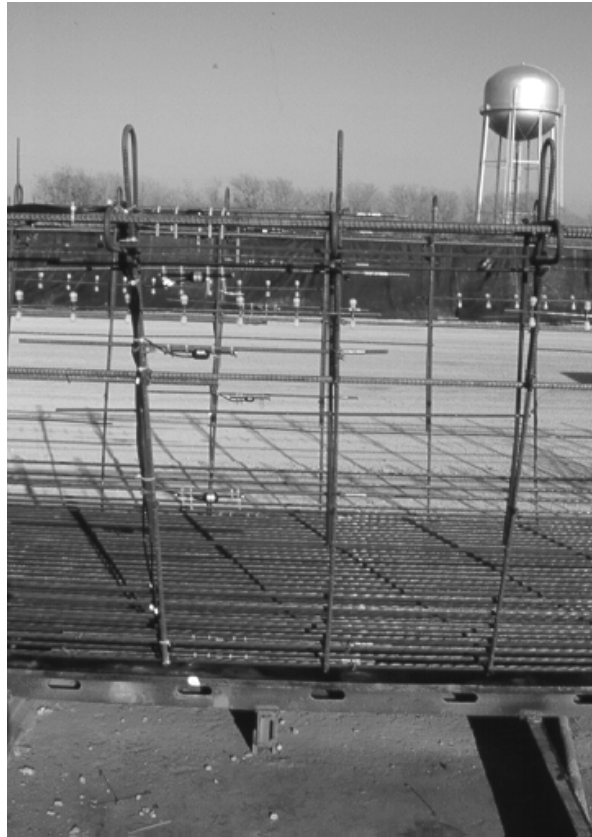
Figure 3.31 - Complete Group of Gauges at Midspan of a Beam
