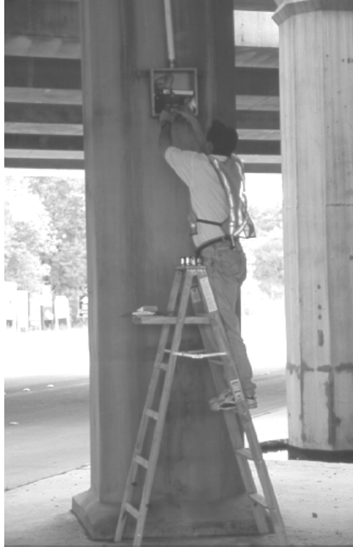
Figure 3.22 - Switching of Batteries and Storage Modules in the Field
