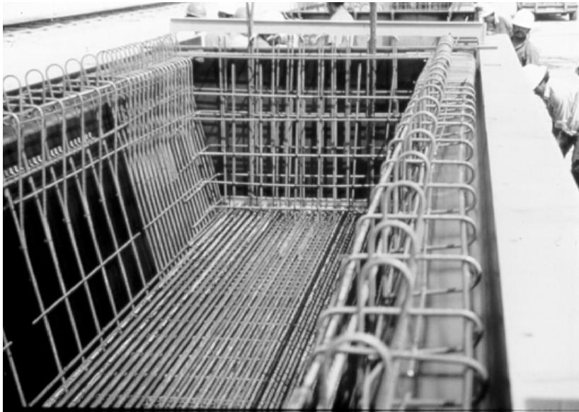
Figure 2.18 - Louetta U-Beam During Fabrication
