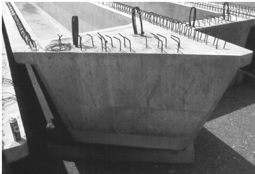
Figure 2.20 - Skewed End Block in a Completed Louetta Beam
