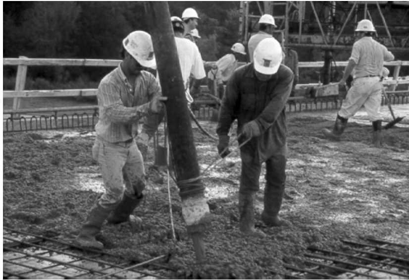
Figure 2.6 - Placement of Louetta Cast-in-Place Deck Concrete
