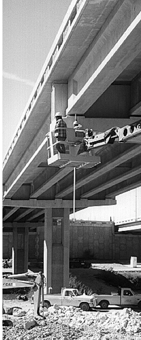
Figure 3.14 - Use of a Man-Lift to Get Surveying Rod to the Level of the Beams in Spans 2, 3, and 4 of the Eastbound North Concho River Overpass
