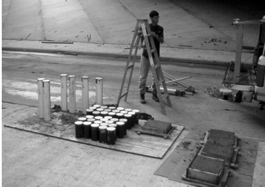
Figure 4.4 - C/S/T Specimens Just After Casting at Jobsite
