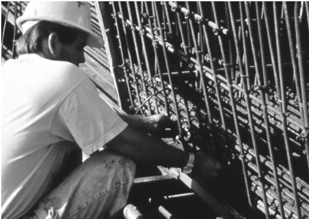
Figure 3.30 - Placement of an Embedded Gauge in a Beam
