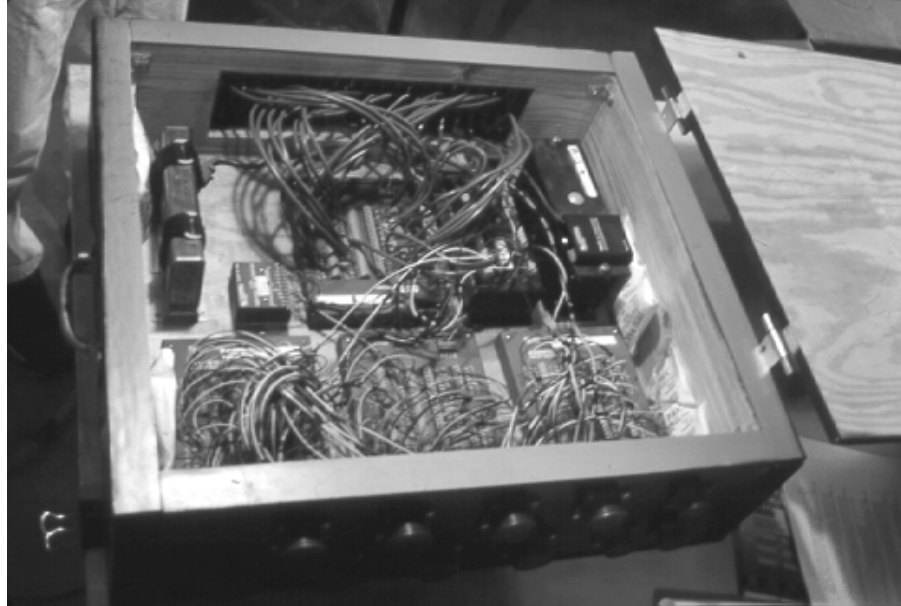
Figure 3.15 - Completed Data Acquisition System (DAS) Box
