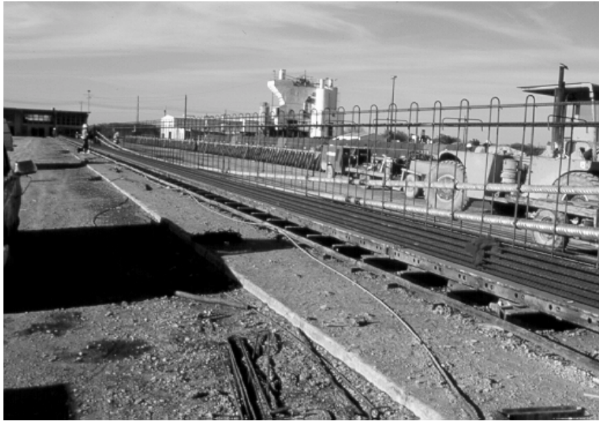
Figure 2.33 - Fabrication of Eastbound HPC Beam
