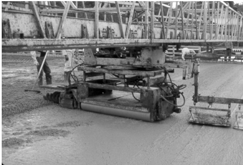
Figure 2.7 - Screeding of Louetta Cast-in-Place Deck Concrete
