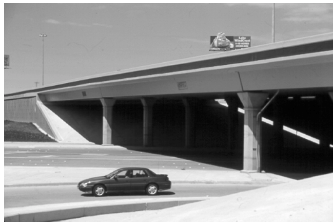
Figure 2.1- Louetta Road Overpass
