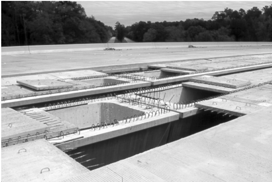
Figure 2.11 - Additional Beams and Panels for Louetta Bridge Widening
