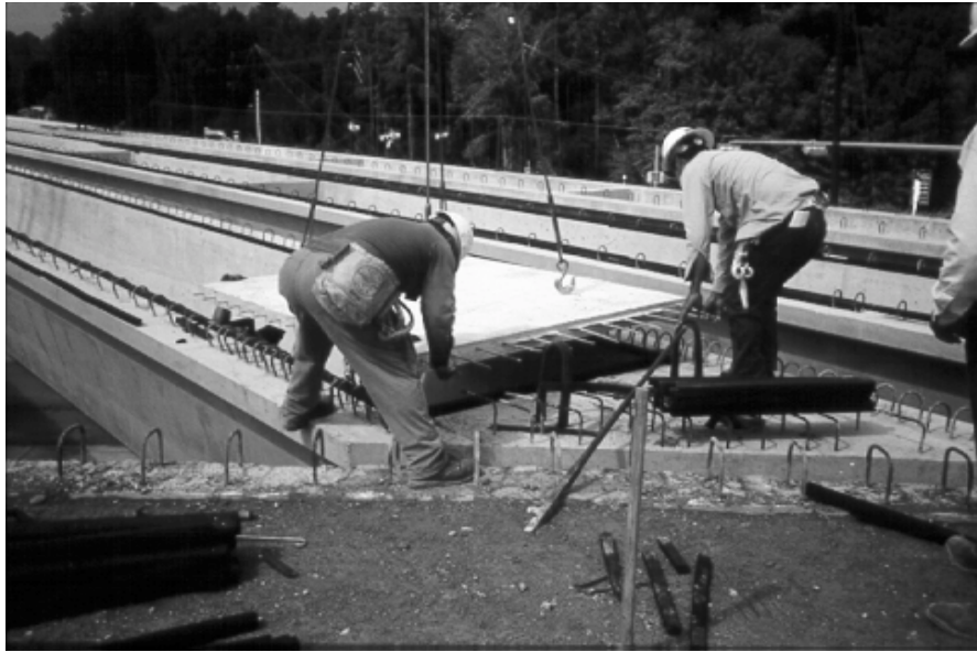
Figure 2.5 - Erection of Precast Panels (Louetta Road Overpass)
