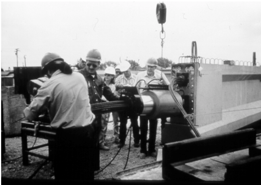
Figure 2.34 - Post-tensioning of Eastbound HPC Beam
