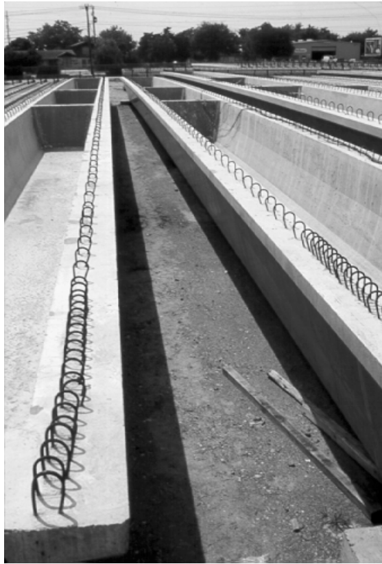
Figure 2.17 - Internal Diaphragms in Texas U-Beam
