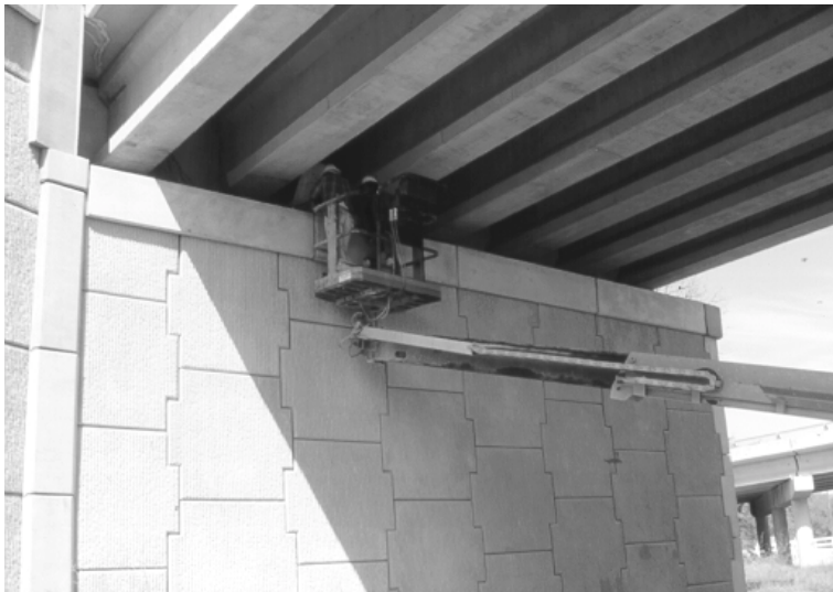
Figure 3.18 - Use of Construction Equipment to Access a DAS Box
