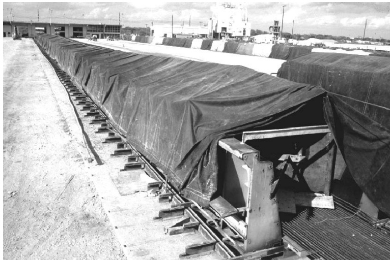
Figure 11.6: Light Steam Curing of U-Beam during Cold-Weather Casting
