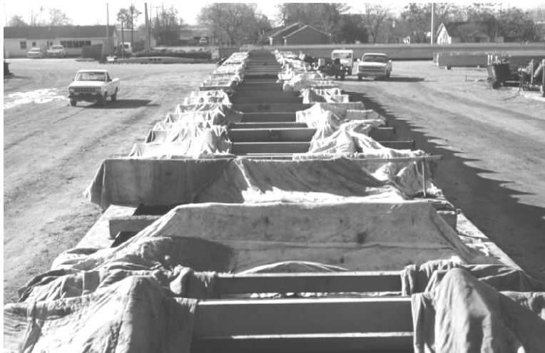
Figure 11.5: Wet Mat Moist Curing of U-beam
