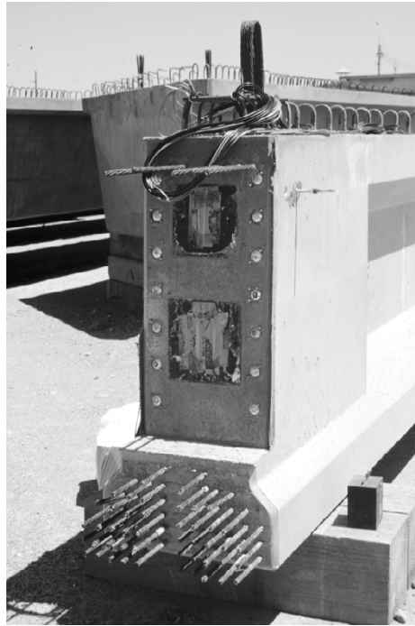
Figure 6.26: North Concho River Overpass AASHTO Type IV Beam
