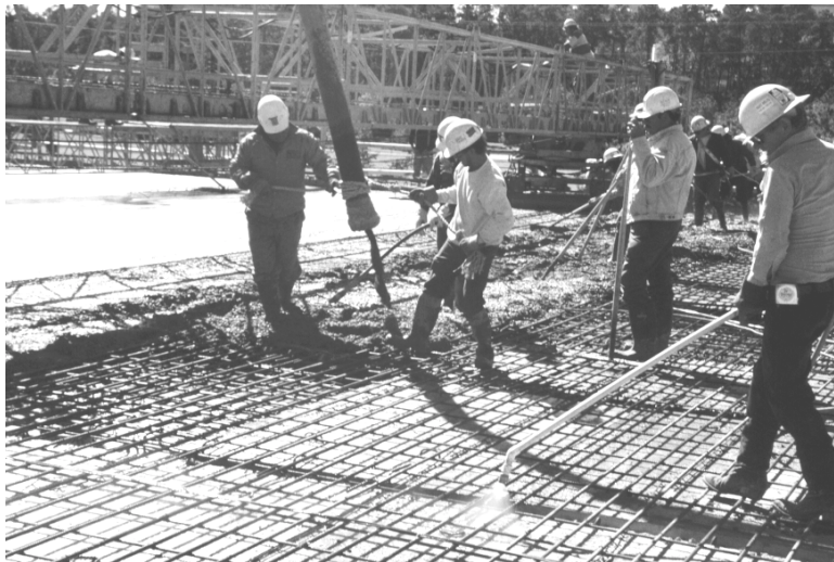
Figure 11.8: Saturation of Deck Panels Prior to Placement of Concrete
