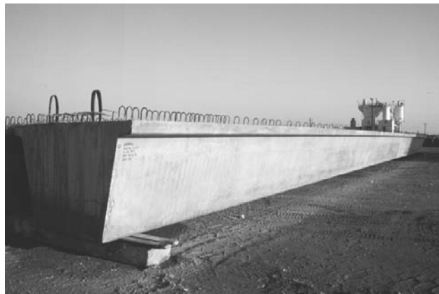
Figure 6.25: Louetta Road Overpass U-Beam
