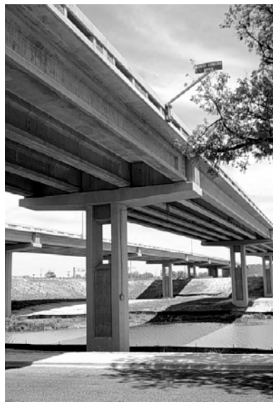
Figure 4.11: North Concho River Overpass Decorative Pier
