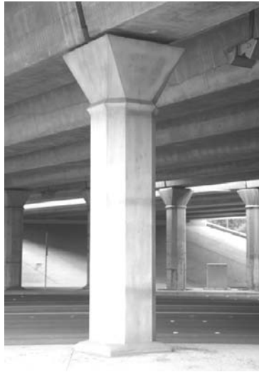
Figure 6.47: Louetta Road Overpass Substructure Element
