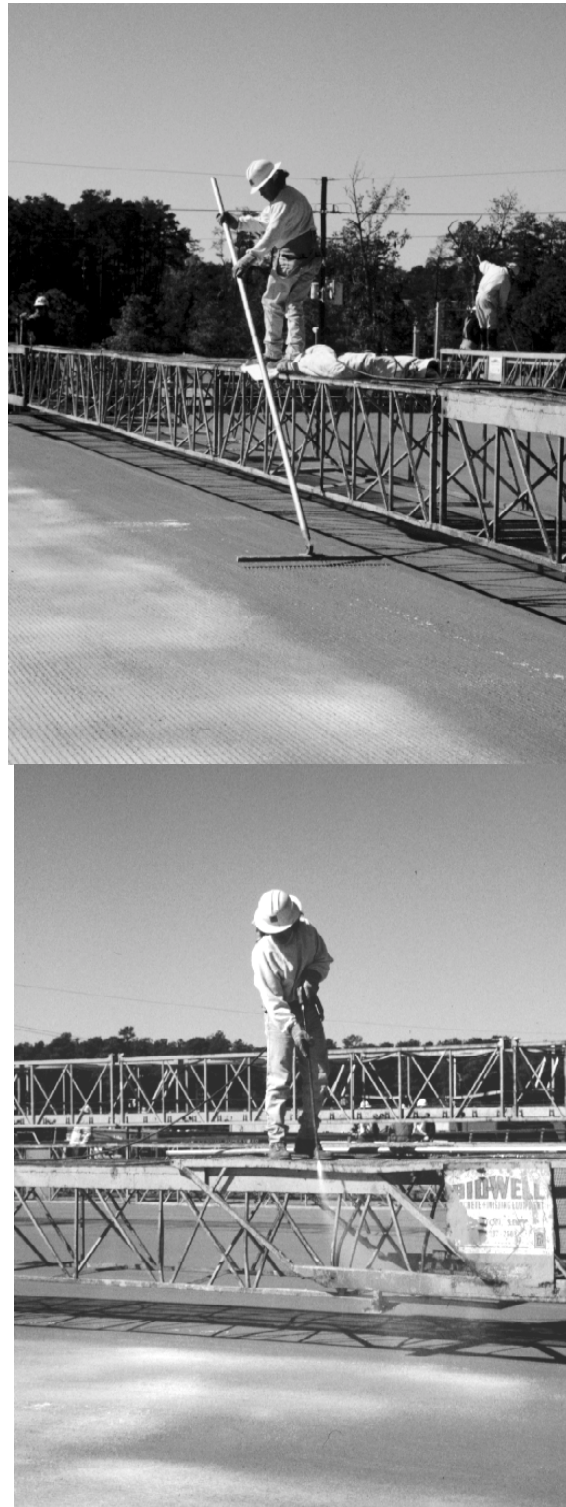
Figure 11.13: Placement of Tining and Curing Compound
