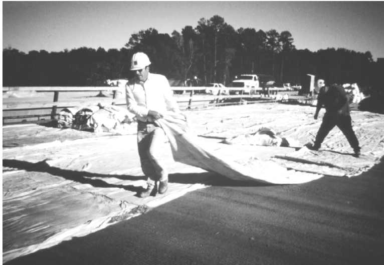
Figure 11.14: Placement of Wet Mats
