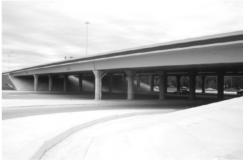
Figure 4.3: Louetta Road Overpass Bridge located in Houston, Texas
