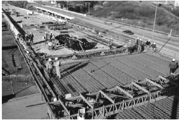
Figure 6.86: North Concho River Overpass Cast-in-Place Deck
