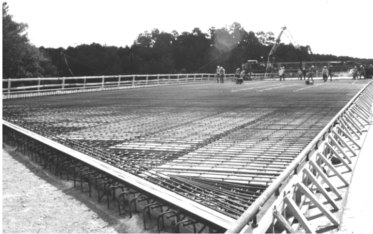
Figure 11.7: CIP Deck Prior to Placement of Concrete
