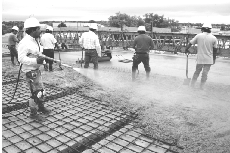
Figure 11.10: Fogging of Concrete throughout Placement and Finishing Operation of Concrete Deck Construction
