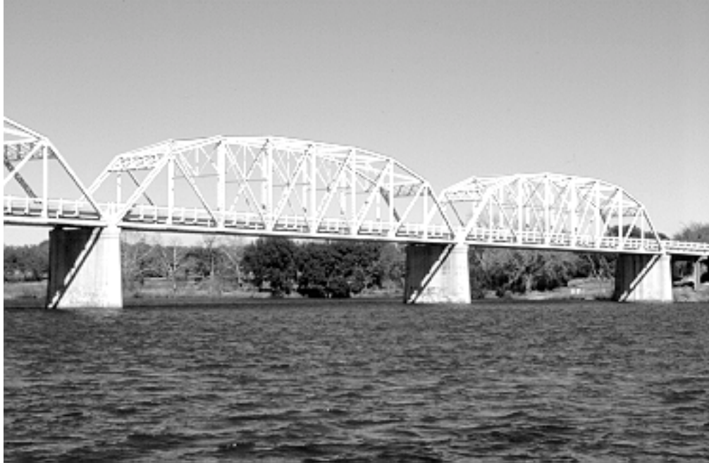
Figure 1.5: Structural Steel Truss Bridge in Buchanan, Texas
