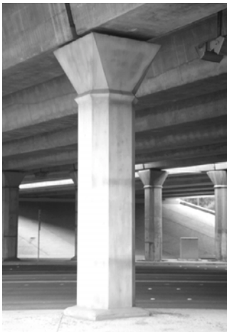
Figure 4.7: Hollow Core Precast Column Element
