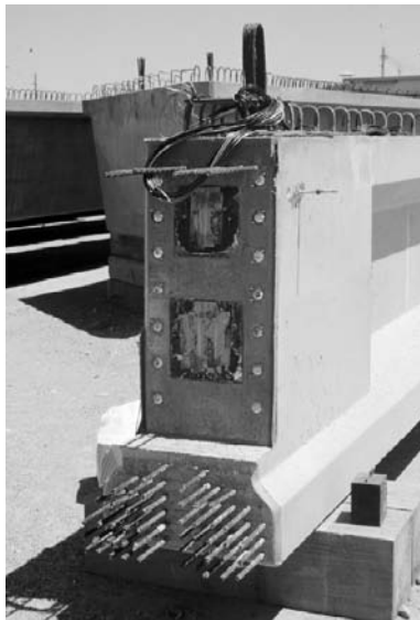
Figure 8.5: North Concho River Overpass AASHTO Type IV Beam
