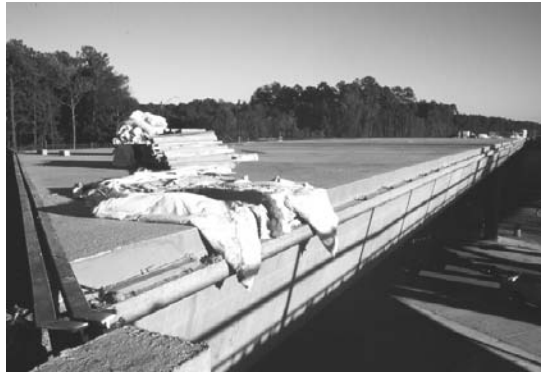
Figure 6.83: Louetta Road Overpass Cast-in-Place Deck
