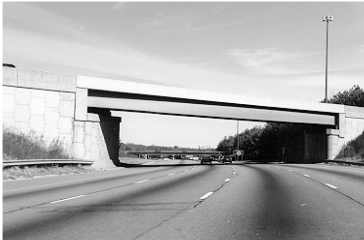
Figure 1.6: Structural Steel Girder Bridge with Composite Concrete Deck in Suwanee, Georgia
