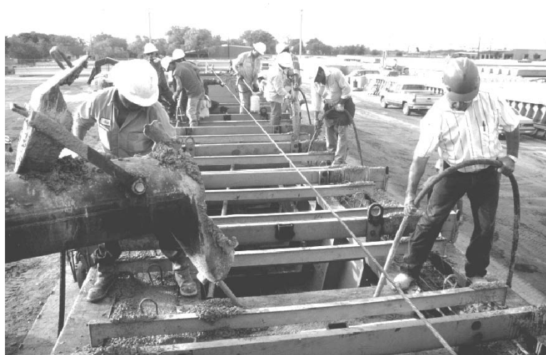
Figure 11.3: Internal Vibration of Concrete for U-beam
