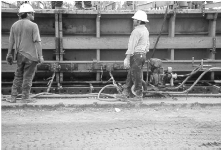
Figure 11.4: External Vibration of Concrete for U-beam
