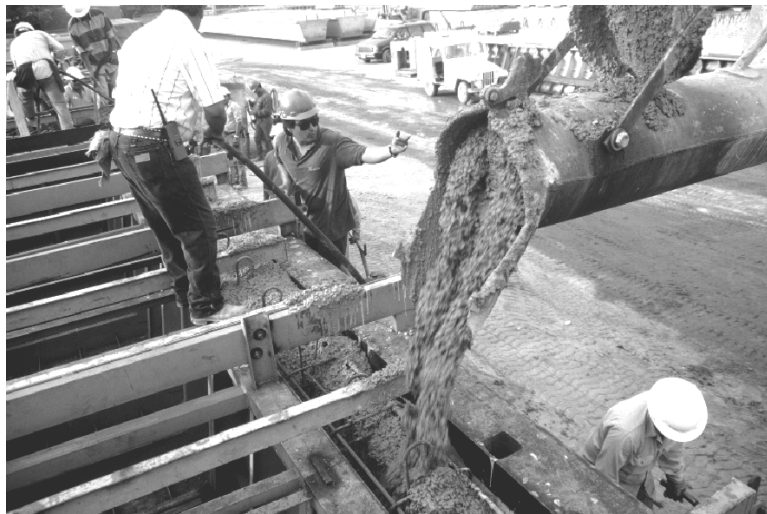
Figure 11.2: Placement of U-beam Concrete
