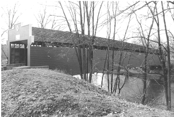
Figure 1.7: Historic Covered Bridge Located in Reading, Pennsylvania
