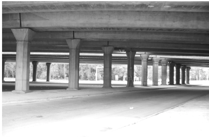
Figure 4.8: Underdeck Perspective of Louetta Road Overpass Bridge
