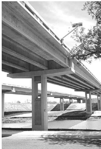
Figure 6.52: North Concho River Overpass Decorative Pier
