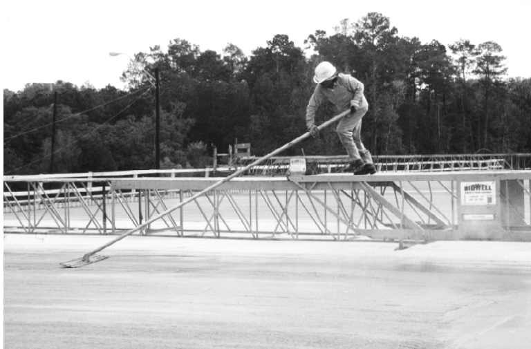
Figure 11.12: Trowel Finish Applied to Fresh Concrete Deck
