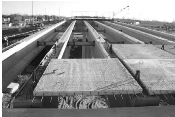
Figure 6.75: North Concho River Overpass Bridge Precast Deck Panels
