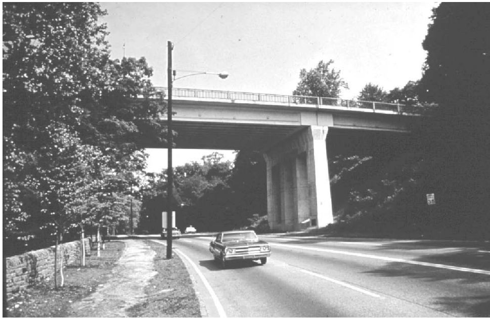
Figure 1.1: Walnut Lane Bridge in Philadelphia, Pennsylvania [103]
