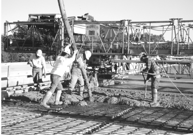
Figure 11.9: Placement of Deck Concrete and Internal Concrete Vibration
