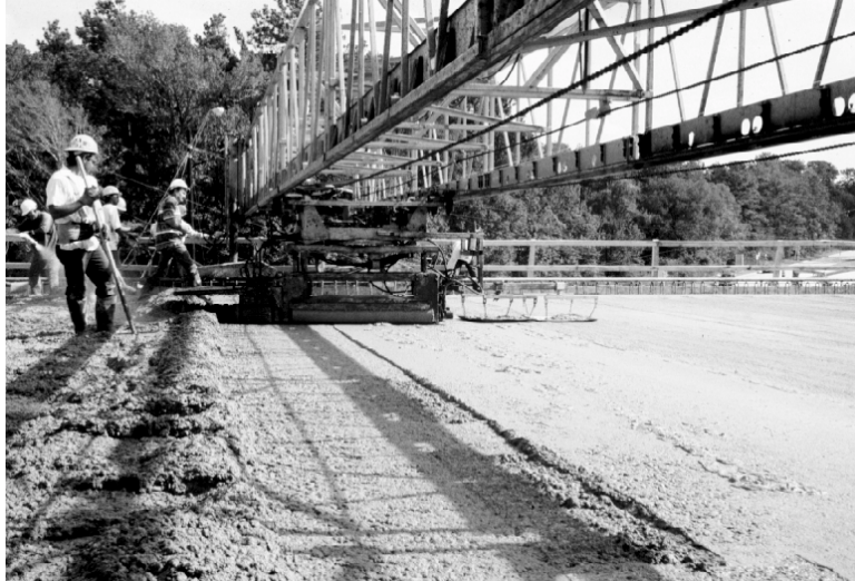
Figure 11.11: Mechanical Spreader Distributes Concrete
