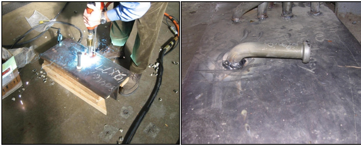
(a) (b) Figure 3.7: (a) Stud Welding (b) Bend Over Test
