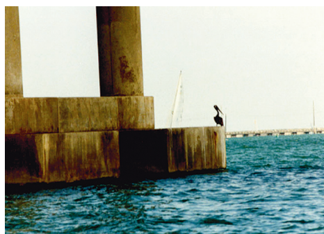
Figure 5 Pelicans, pigeons, and boats may contribute to premature anode deterioration.
