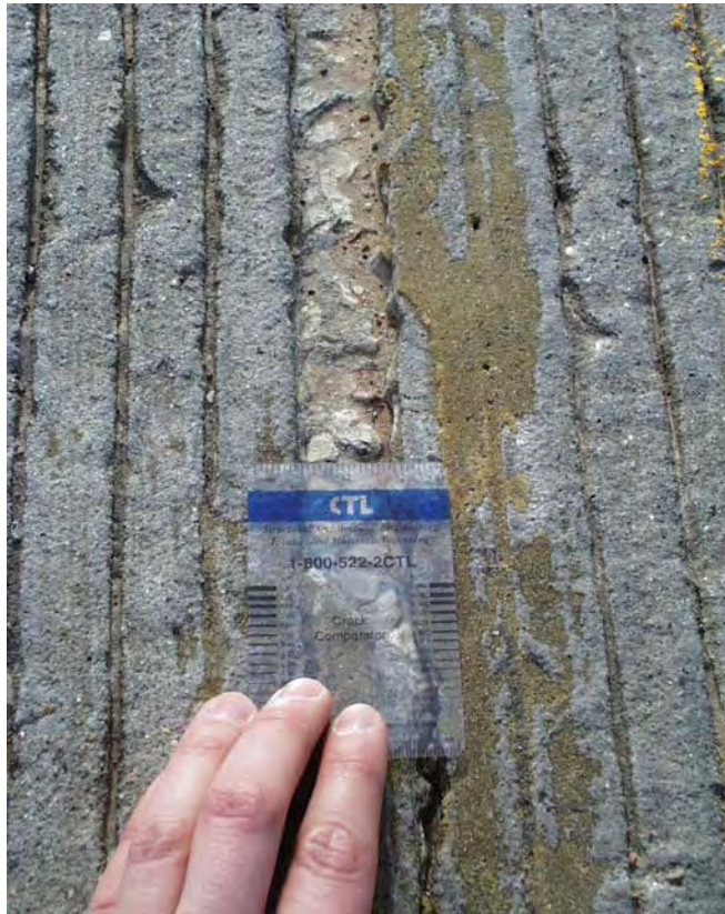
Figure 5.1 Close-Up of Crack in Louetta Southbound Deck
