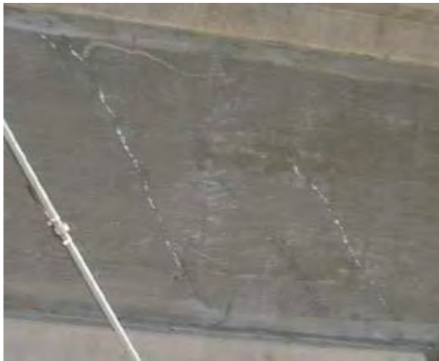
Figure 9: Underside of Cracked Panel in Louetta Bridge
