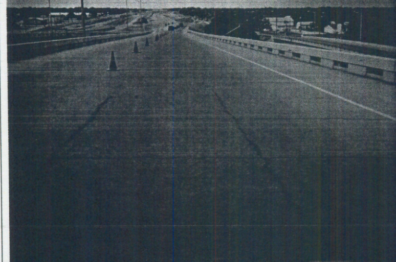
Photo 8: View of the westbound bridge, the western end of Span 4 showing the rectangular cracking pattern.
