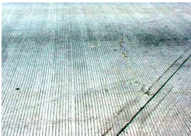
Figure 7: Another Large Crack in Louetta Bridge Deck (Contrast Raised to Highlight Crack)
