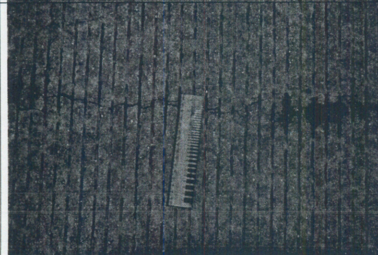
Photo 6: Closeup view of a longitudinal crack.
