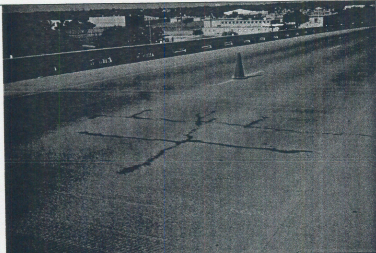
Photo 7: View of the eastbound bridge, the western end of Span 5, showing cracking pattern at the edge of span.
