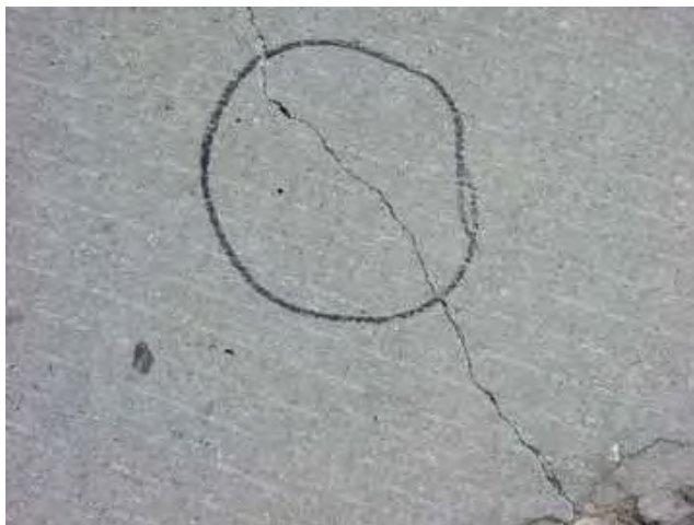
Figure 3: Region of Cracked HPC Deck Used for Chloride Determination
