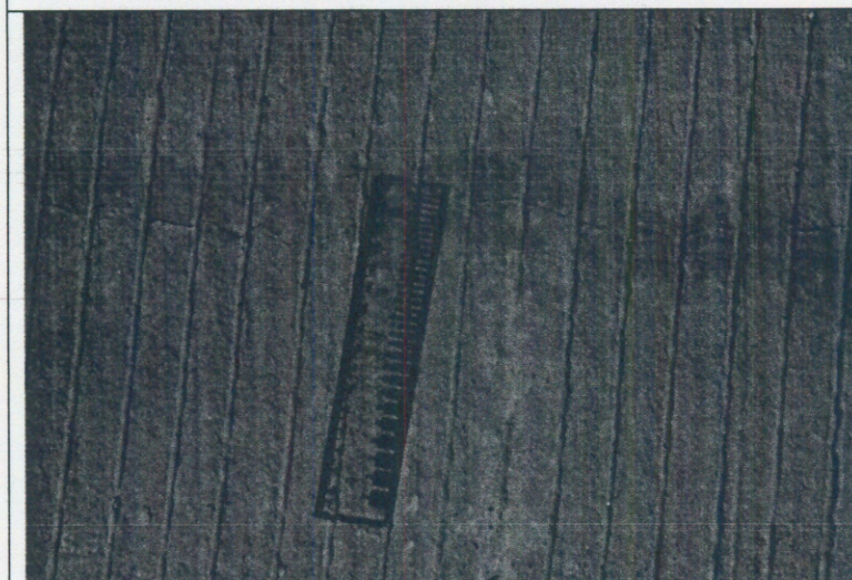
Photo 7: View showing typical crack in the bridge deck. Crack width is less than 0.031 in. and is categorized as hairline.
