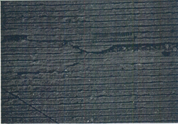
Photo 8: View showing spalling associated with cracks in the deck at span ends.
