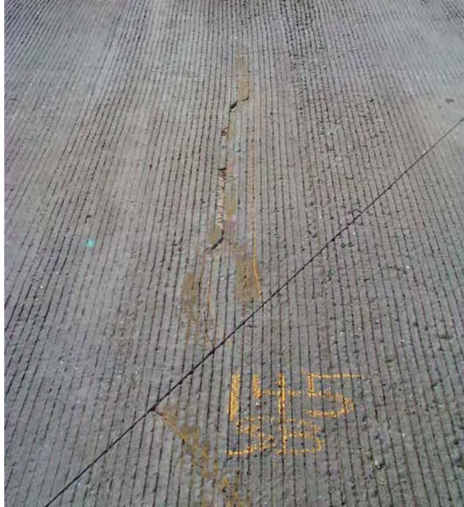
Figure 5.2: Severe Crack in Louetta Southbound Deck
