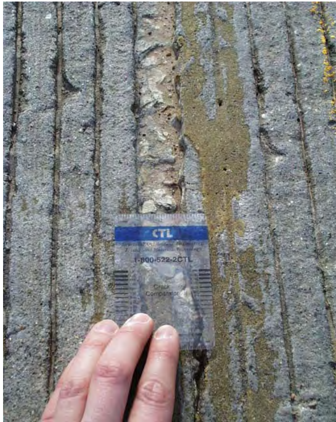
Figure 5.1: Close-Up of Crack in Louetta Southbound Deck
