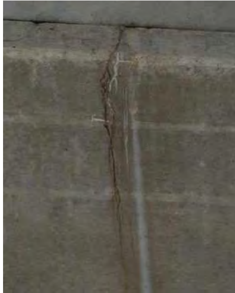
Figure 8: Large Crack in Flange and Web of Louetta U-Beam
