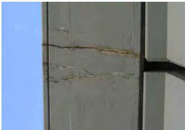
Figure 10: Cracked Soffit Section on Westbound Deck
