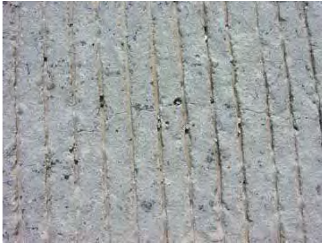
Figure 5: Longitudinal Cracks in the Amarillo Creek Bridge
