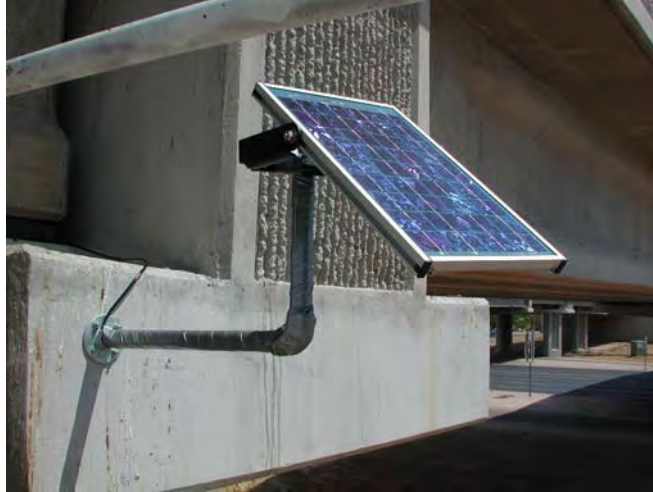
Figure 3.8: Solar Panel Mounted on San Angelo Bent Cap
