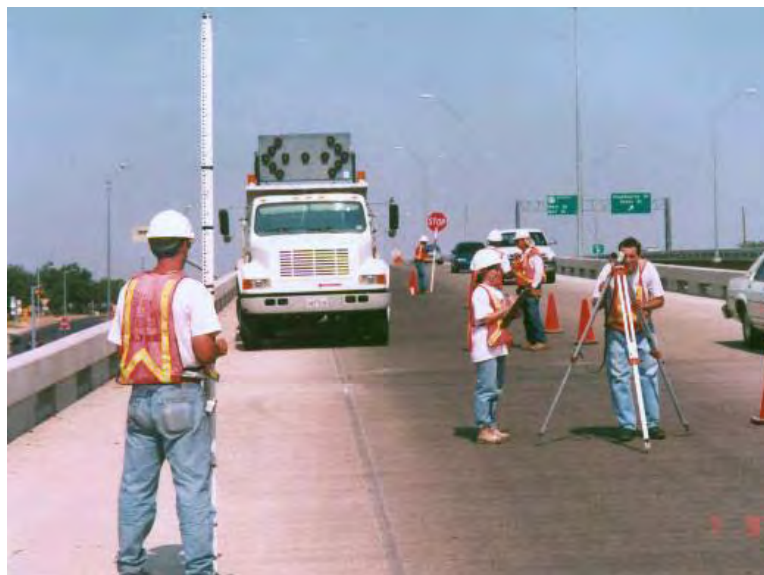
Figure 4.5: Camber Measurements at San Angelo
