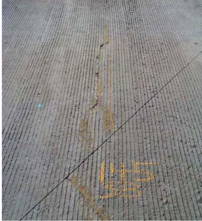
Figure 5.2 Severe Crack in Louetta Southbound Deck
